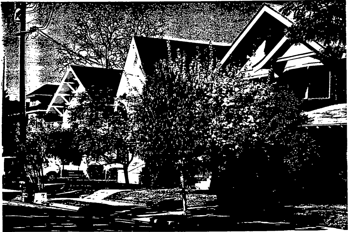
3 story historic homes abutting the property at 2362 W. Washington Blvd.
