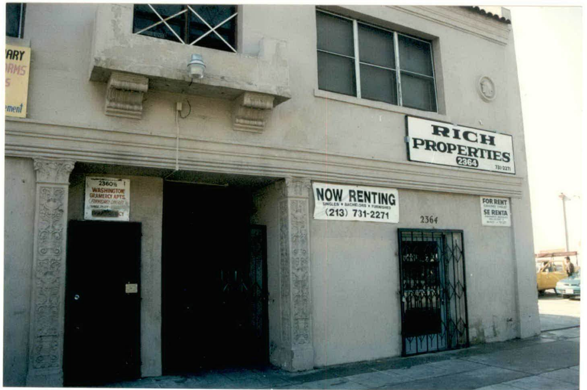
2362 (2360-2364)W. Washington Blvd., Rich Properties, site of Nextel's proposed unmanned facility and 12 roof-top antenna installation on penthouse visible on roof. Note For Rent (213) 731-2271 signs. Residential apartments available in building.
