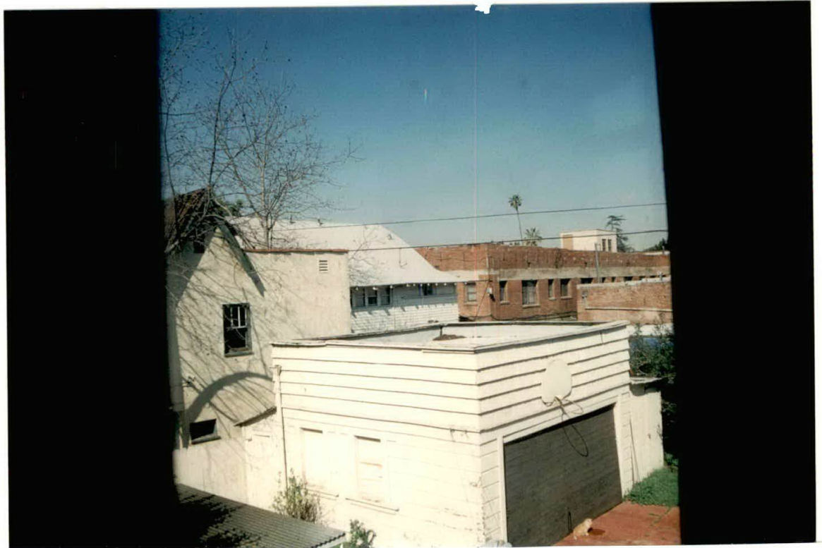
View of 2362 W. Washington Blvd. (brick building with penthouse), site of Nextel's proposed unmanned facility and 12 roof-top antenna installation, from adjacent residential property on 20 th Street.
