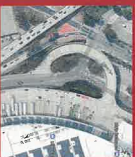
New Street Ramp 08/22/2025 *
