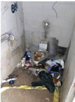
Boardwalk Public Restrooms 2020-03-12 at 6.04.02 PM.png 502K
