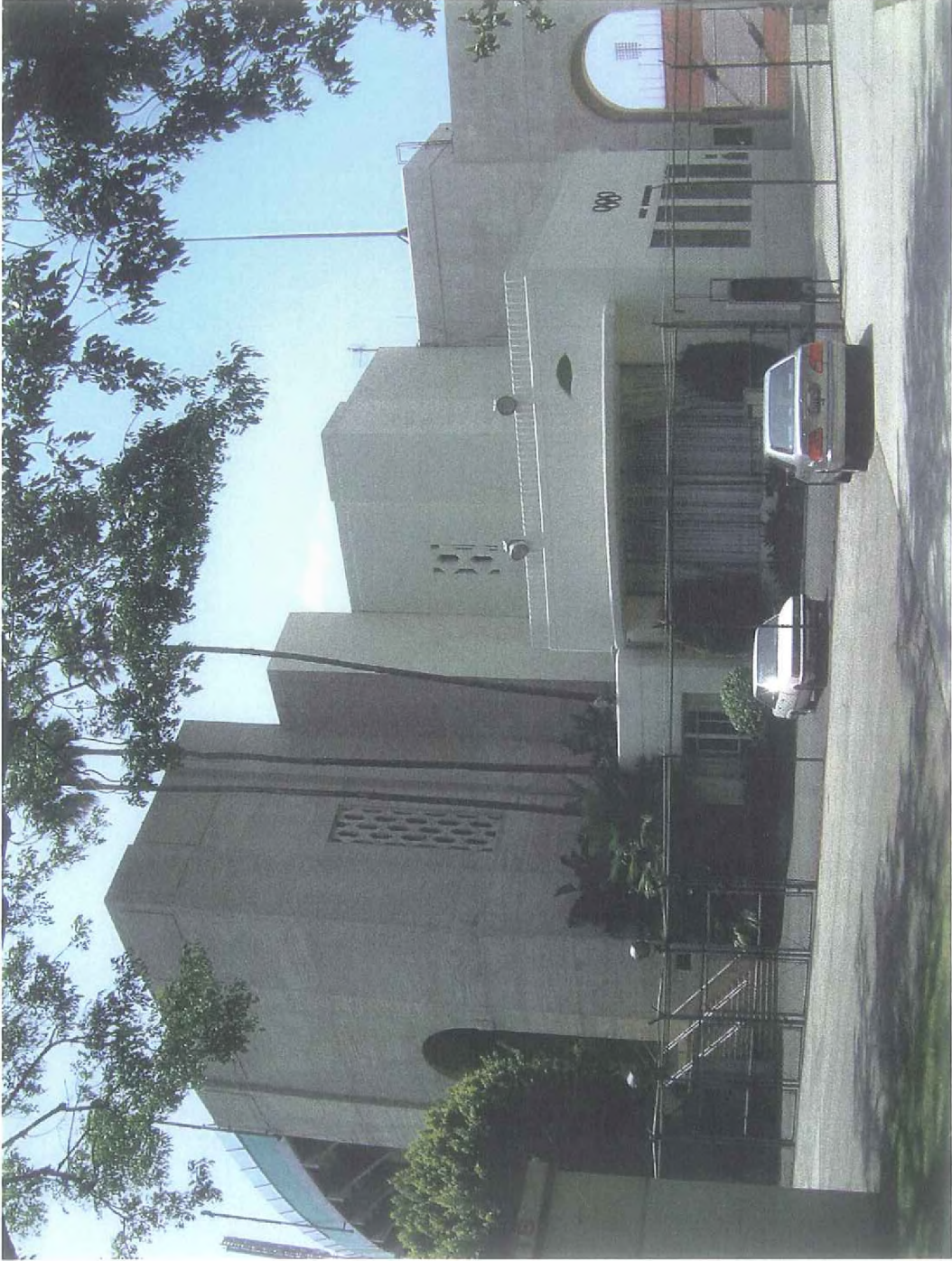
Exterior View of South Peristyle End
