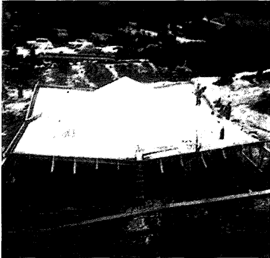
James F. Real Studio-Office, freshly poured concrete roof (Pacific Bridge Company photo)
