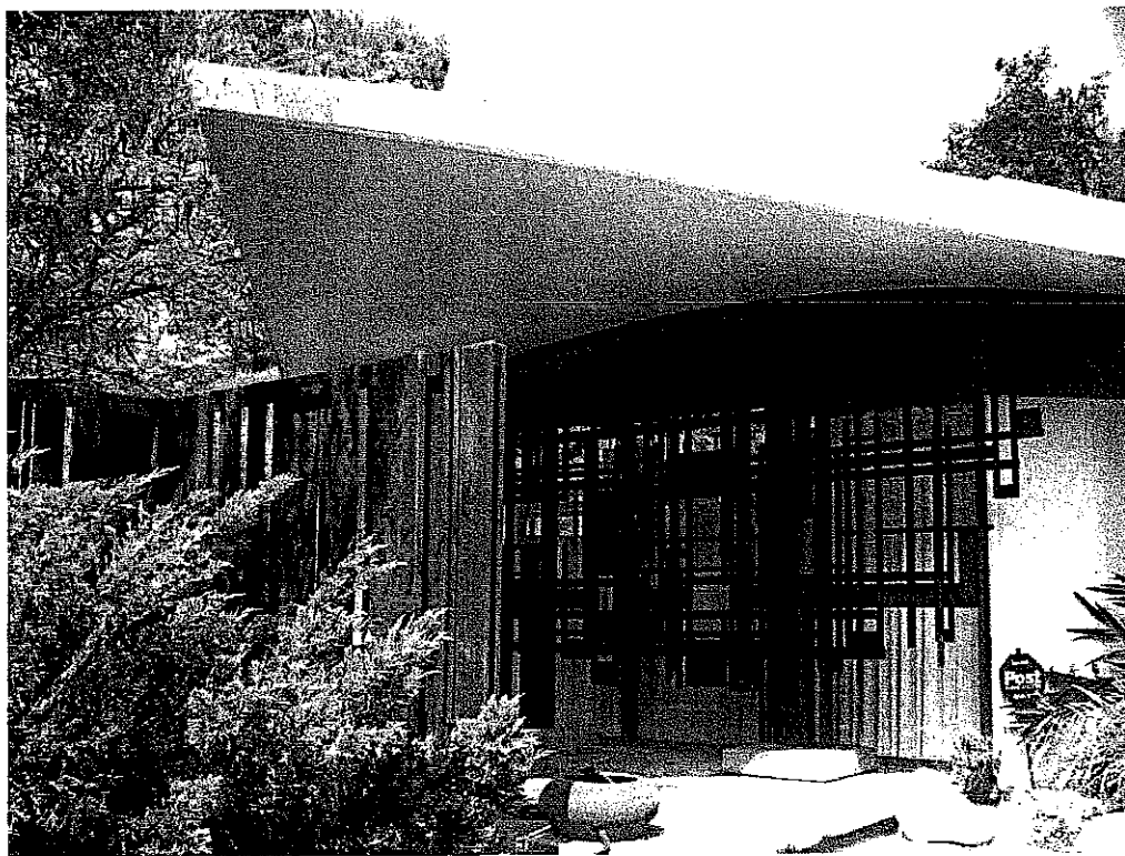
James F. Real Studio-Office, front porch, 77 Patrician Way (Photograph by Charles J. Fisher)
