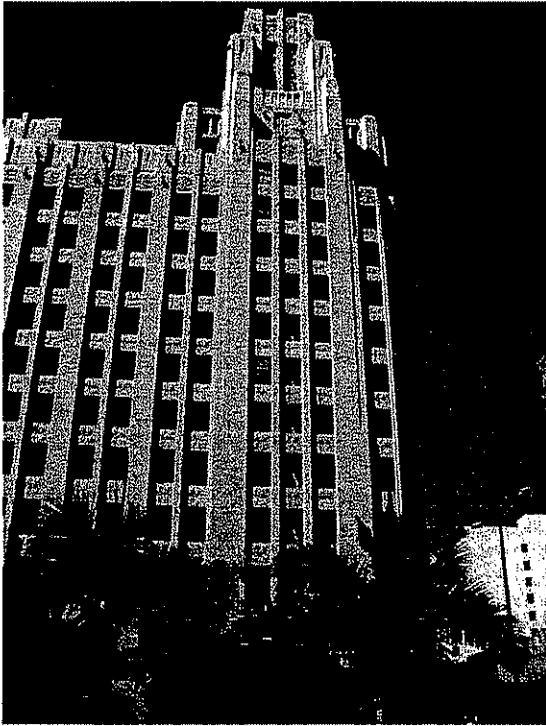
Photo #1: West elevation, Title Guarantee Building after restoration of terra cotta façade, window restoration, and maintenance of original, internal fire escape.
