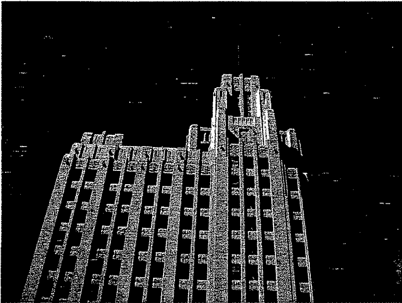
Photo #2: Upper façade of Title Guarantee Building after restoration.
