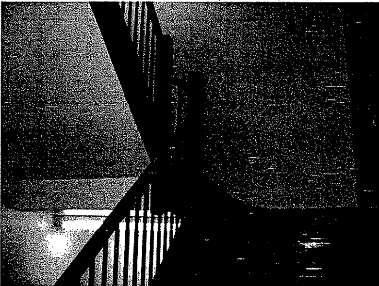
Photo #58: Internal stairwell and fire exit. Walls were painted, but staircase left "as-is" for continued exiting function.
