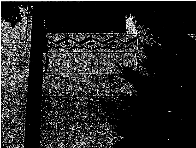
Photo #12: Terra cotta on west elevation. Any cracked or damaged pieces were replaced, and surface was reglazed to provide uniform appearance.
