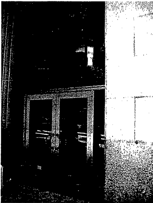
Photo #18: Entrance doors, cleaned and repaired.
