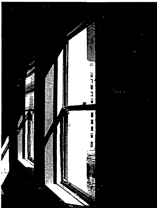
Photo #38: Original steel 1/1 windows on all facades were restored. Most are in operable condition.
