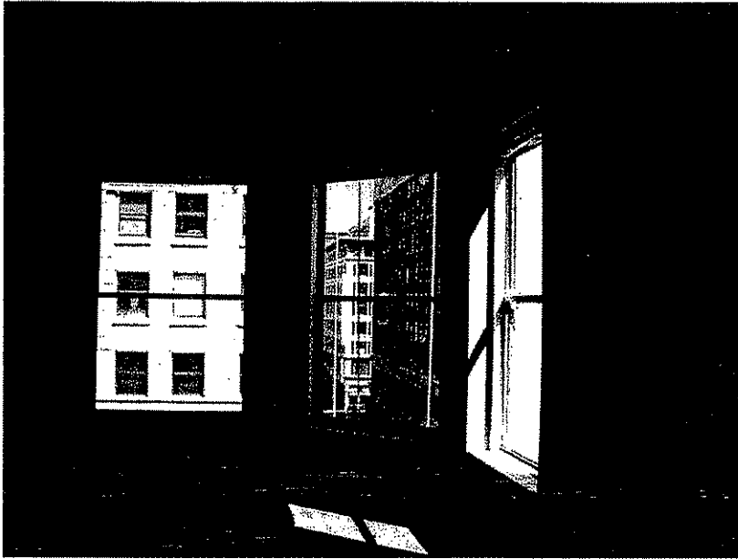
Photo #39: Original steel, 1/1 windows on all facades were retained and restored. Most are in operable condition.
