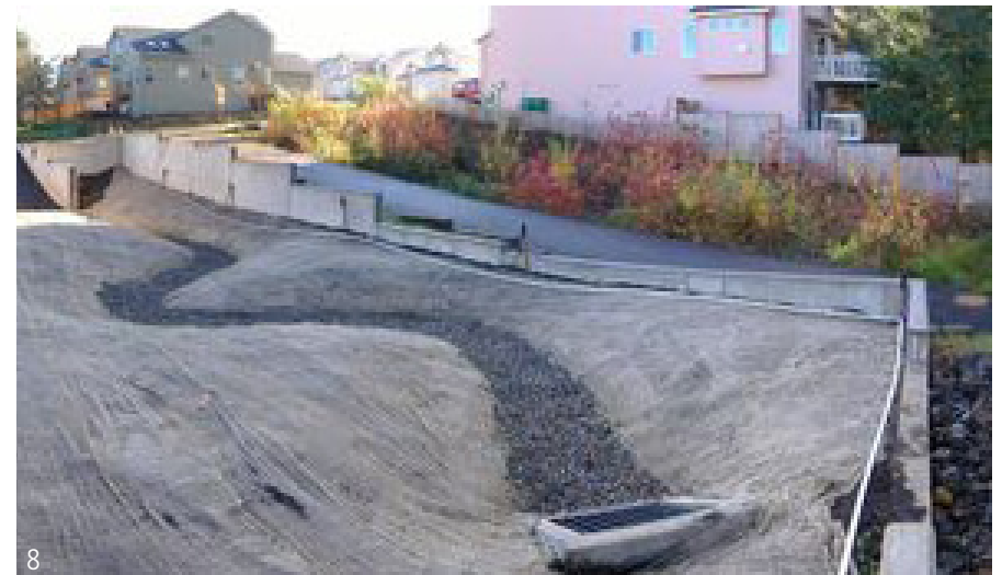
Bioswale - under construction (foreground), completed (background)
