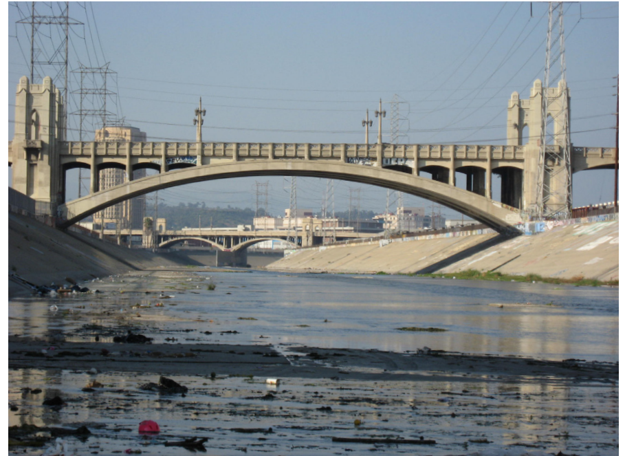
LA River, Downtown. View of 4th Street and 1st Street bridges
