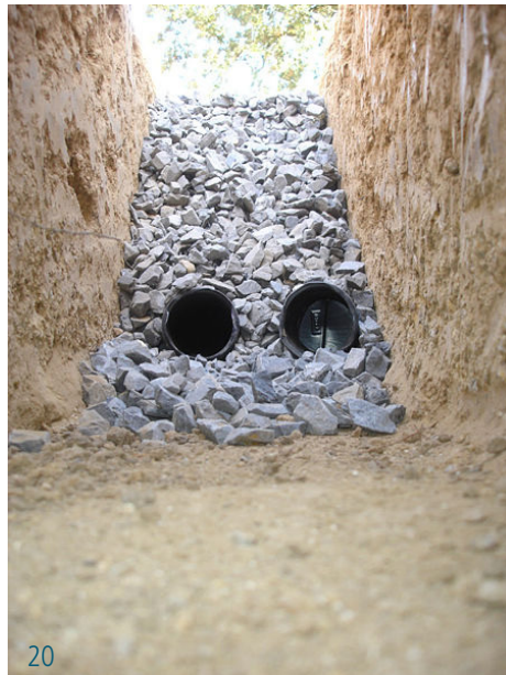
French drain under construction
