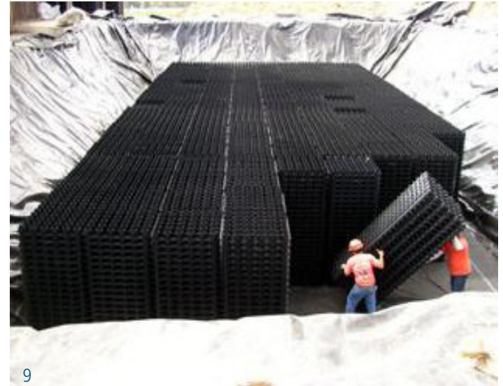
Cistern under construction
