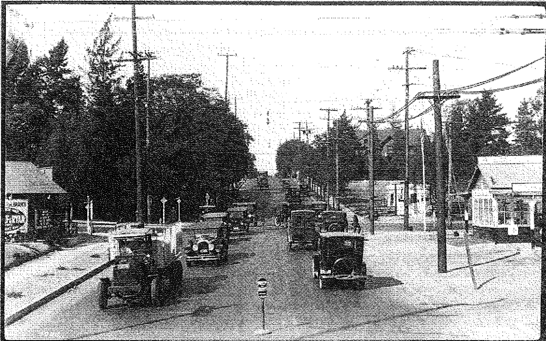
View of Western Avenue from Adams Boulevard, just north of the district, 1924
