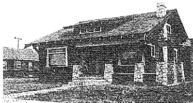
ELMER CALIFORNIA COTTAGE WITH TYPICAL WINDOW ARRANGEMENT IN THE PORCH AND WITH PROMINENT PORCH BRICK AND CHIMNEY OF BRICKWORK.
