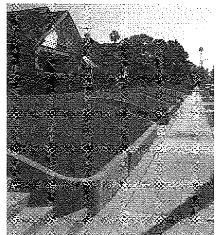
Historic retaining walls often comprised of concrete or Arroyo Stone, are an important part of the neighborhood setting
