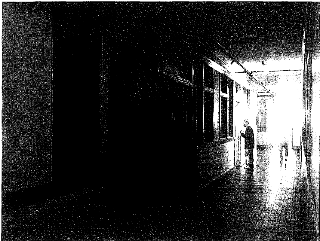
Spreckels Building, upstairs hallway, 714 S. Hill Street, December 2, 2009 (Photograph by Charles J. Fisher)
