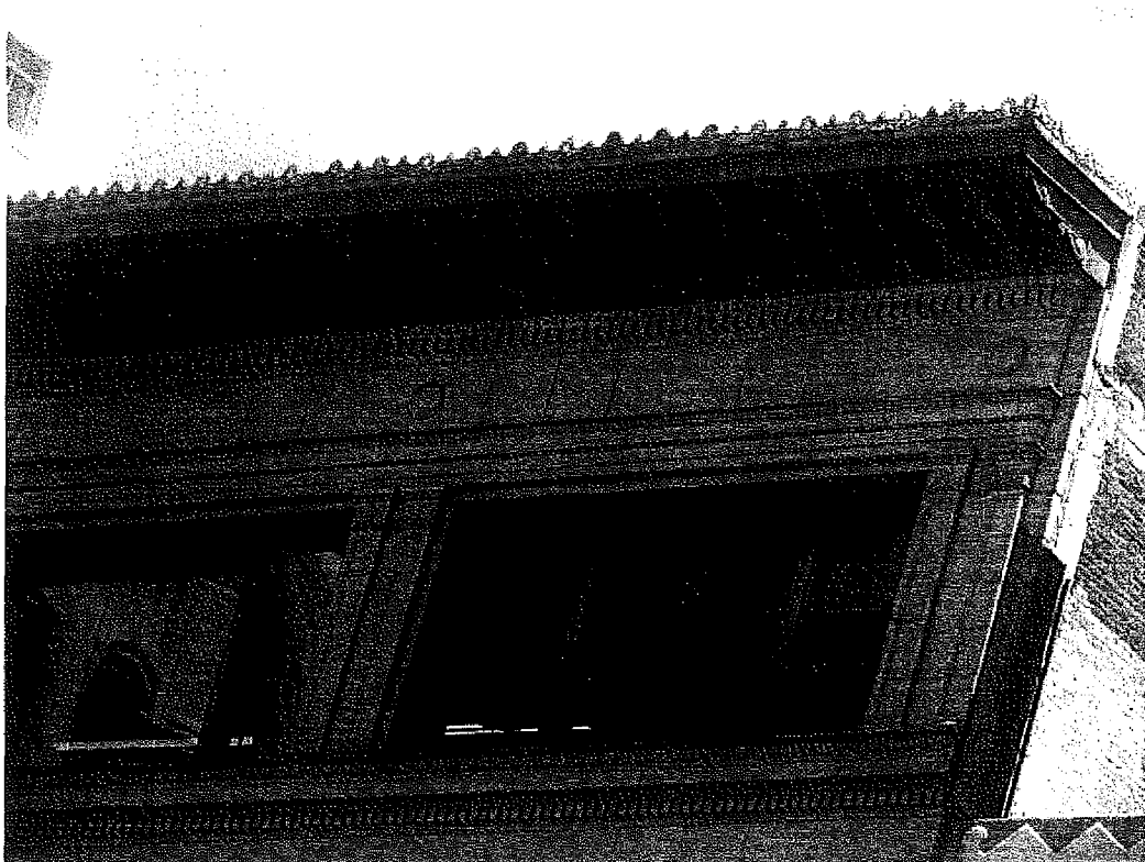
Spreckels Building, cornice, 714 S. Hill Street, June 2, 2009 (Photograph by Charles J. Fisher)
