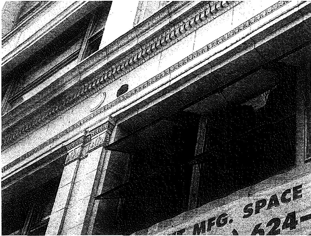
Spreckels Building, transom windows, 714 S. Hill Street, June 2, 2009 (Photograph by Charles J. Fisher)
