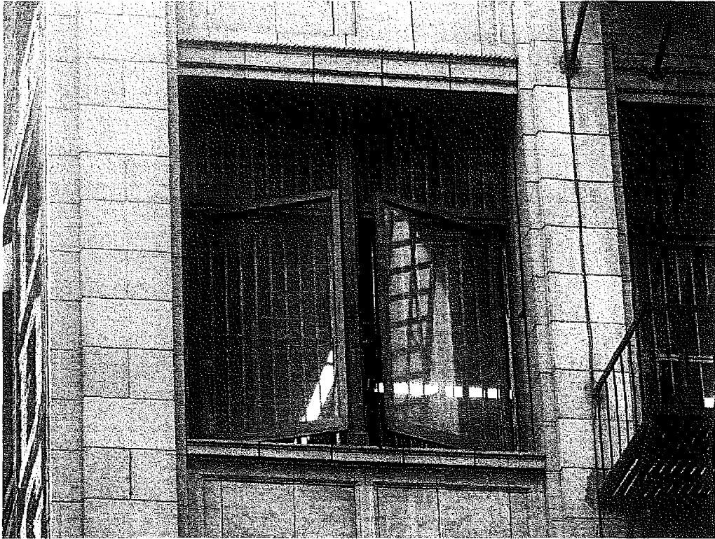
Spreckels Building, casement windows, 714 S. Hill Street, June 2, 2009 (Photograph by Charles J. Fisher)
