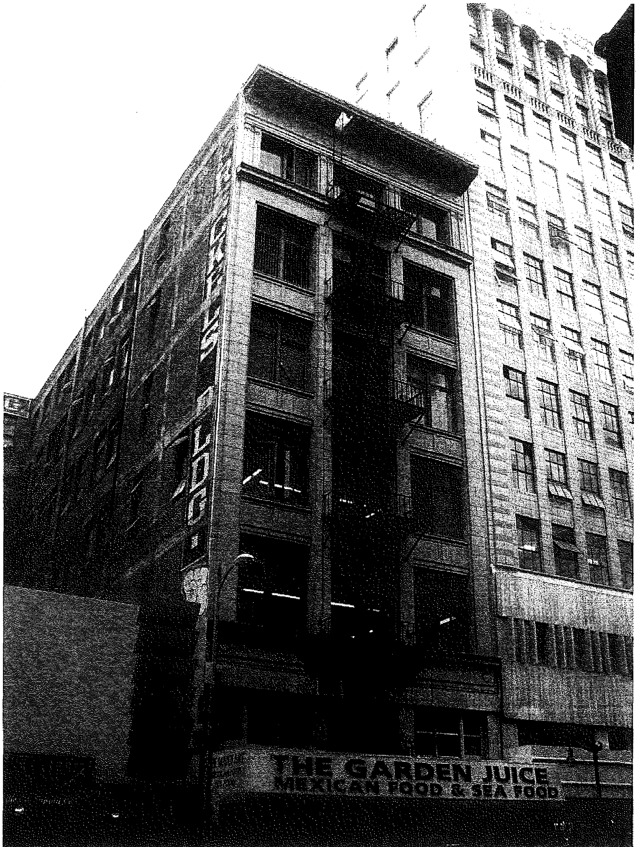
Spreckels Building, 7 th Street facade, 722-24 W. 7 th Street, June 2, 2009 (Photograph by Charles J. Fisher)
