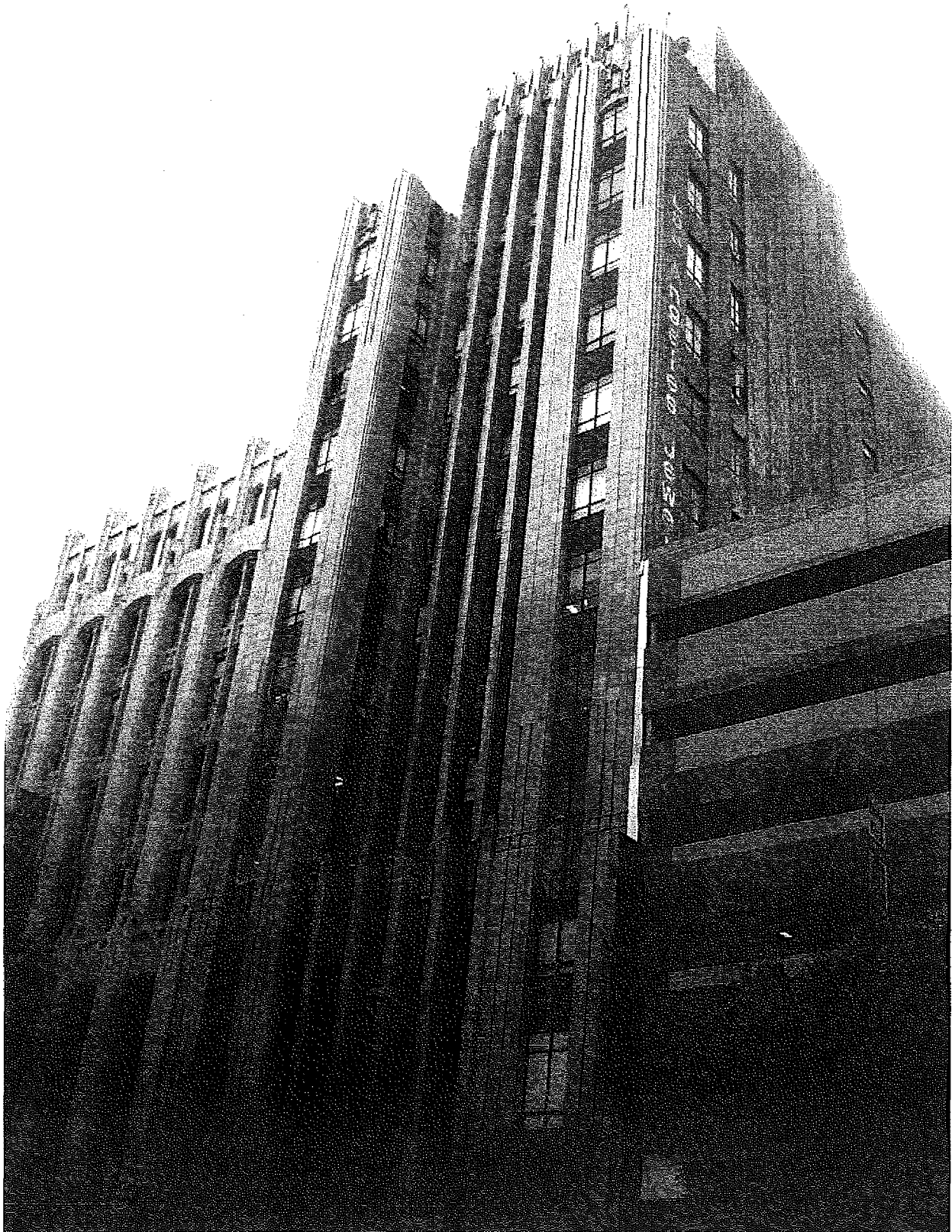
Sun Realty Company Building, 629-33 S. Hill Street, May 29, 2009 (Photograph by Charles J. Fisher)
