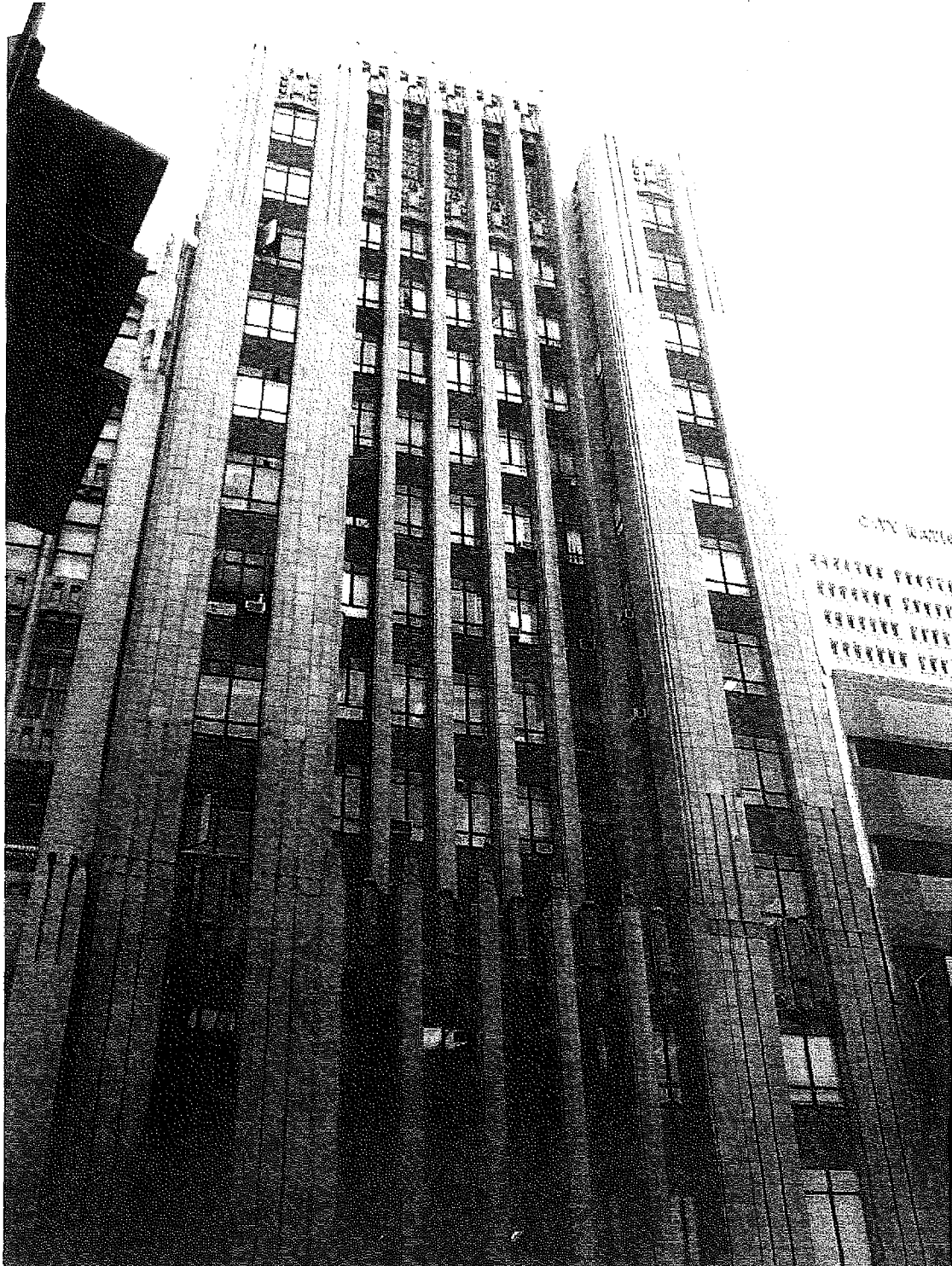
Sun Realty Company Building, 629-33 S. Hill Street, May 29, 2009 (Photograph by Charles J. Fisher)
