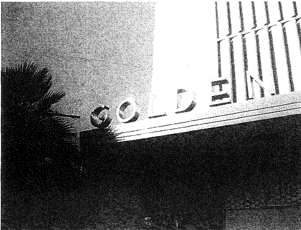
6. Golden State Mutual Life Insurance Company Home Office, entrance canopy detail with stainless steel fascia and edge lettering spelling "GOLDEN STATE MUTUAL LIFE". View: NE
