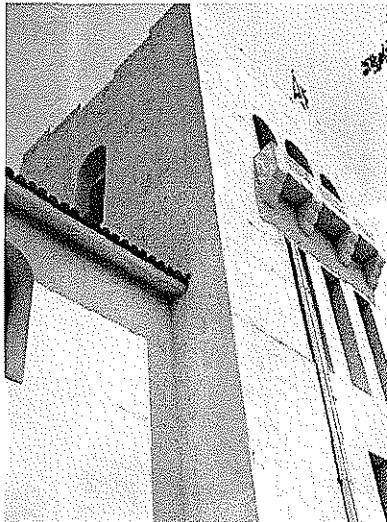
HR018 - Caracol Tower: south façade
