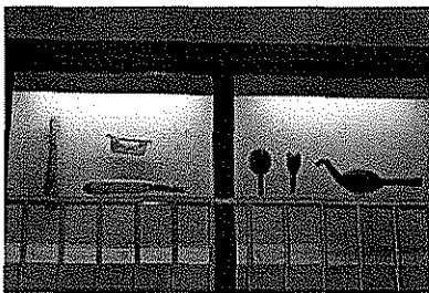
E020 - Inconsistent display case lighting typical throughout
