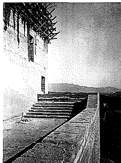
H007 - C arcoal tower & south terrace under construction
