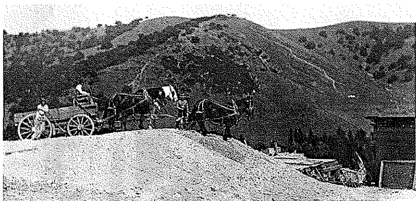
H006 - Under construction May 1913
