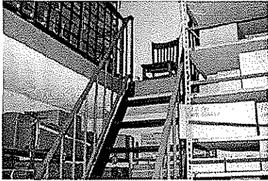
HR024 - Caracol 7; Mezzanine stair
