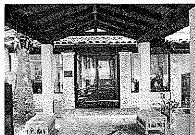
HR003 - Upper entrance vestibule, added 1941, and walkway canopy c.1977
