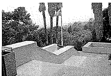
HR006 - South entrance terrace; West End
