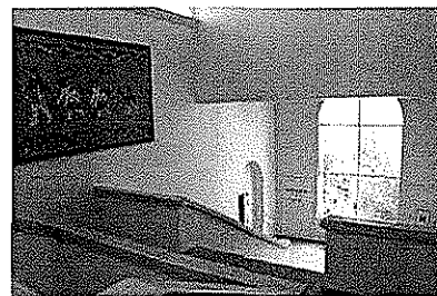
HR011 - Main stair (current condition)
