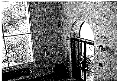
HR013 - Monumental window & door to terrace at lower lobby
