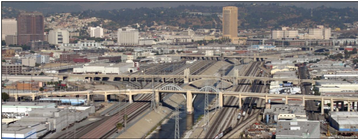
Figure 16 Aerial Views of 6 th Street Viaduct
