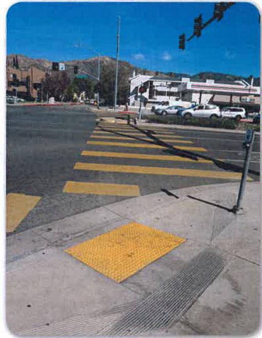
Figure 17 - Ramps with Rumble Strips
