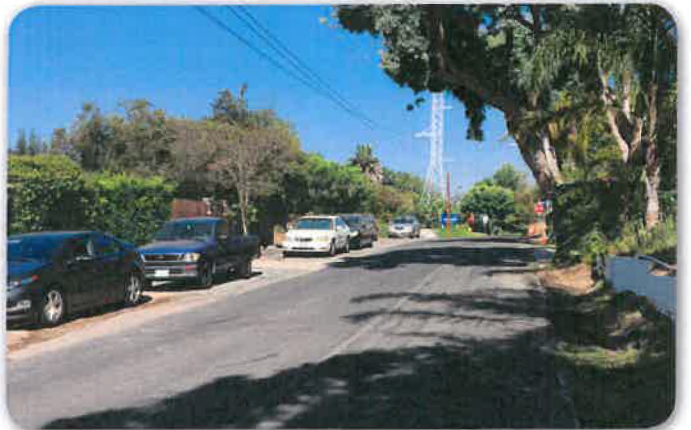
Missing Sidewalk along Waverly Drive (looking West)
