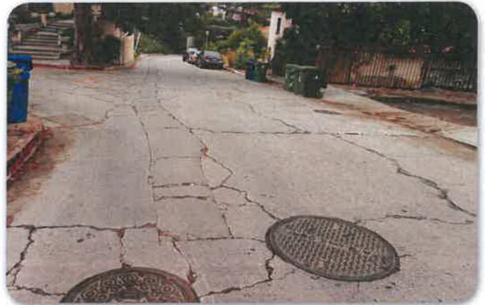
Utility hole coverings on Angus Street
