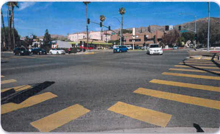
Figure 16 - High visibility crosswalks
