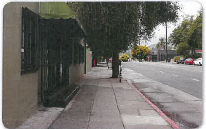
Rowena Avenue Southside Sidewalk (looking West)
