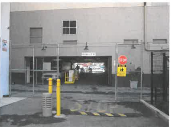
View 8: Vehicle access crossing.
