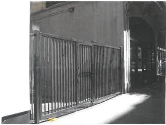
View 9: Looking at alley entrance from 5th Street.
