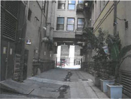
View 3: Looking northeast along alley toward 4th Street entrance.
