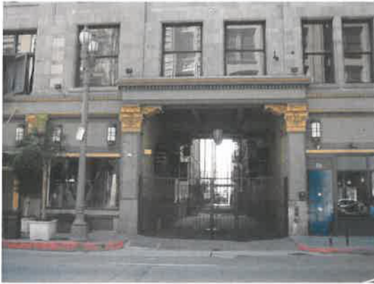
View 1: Looking at alley entrance from 4th Street.
