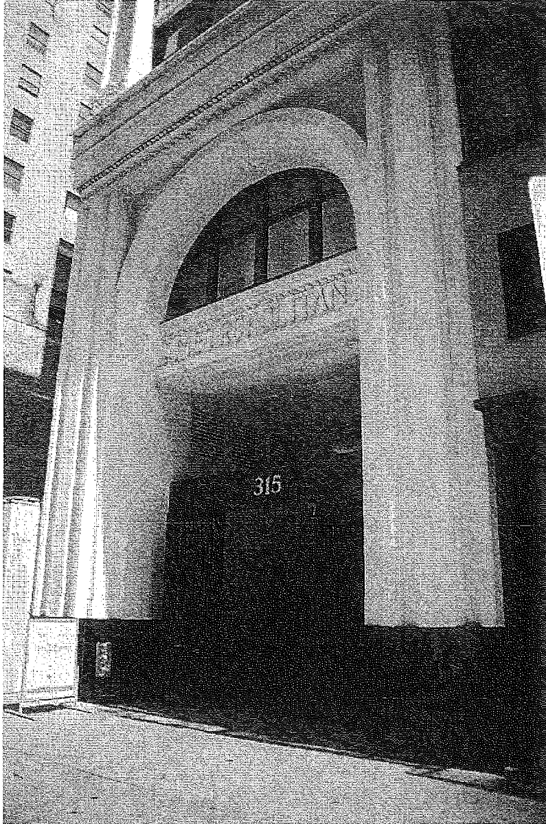
Photo 3. Metropolitan Building, residential entrance, view northwest (Chattel, 2011).
