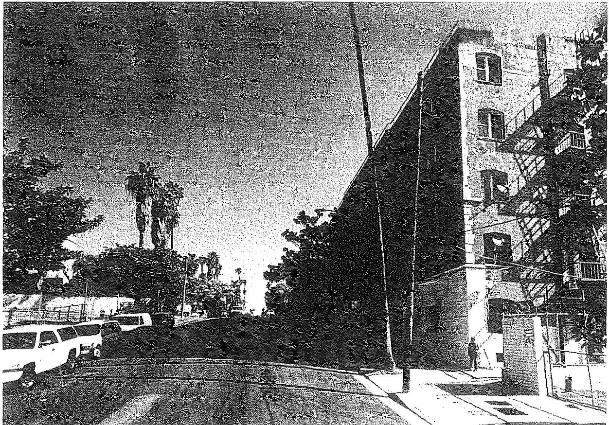
6. VIEW OF EAST SIDE OF HOBART BOULEVARD OPPOSITE PROJECT SITE
