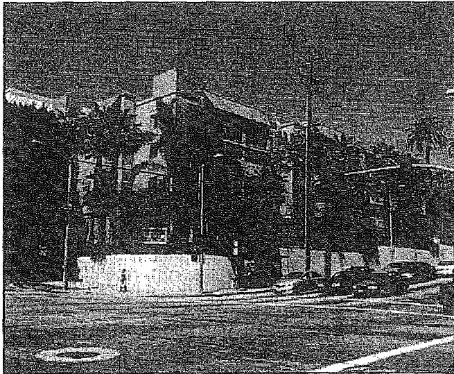
View 10: St. John of God Retirement Center west across Western Avenue from the on-site Golden State Building.
