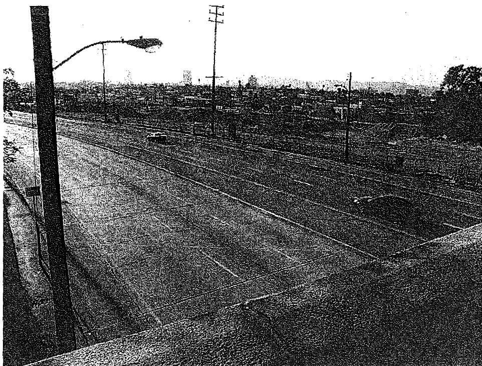
FACING NORTH, PHOTO TAKEN FROM WEST SIDE OF BRIDGE PRIOR TO COMPLETION OF LOWE'S STORE, FORMER SITE OF VINEYARD POWER STATION AND SEARS
