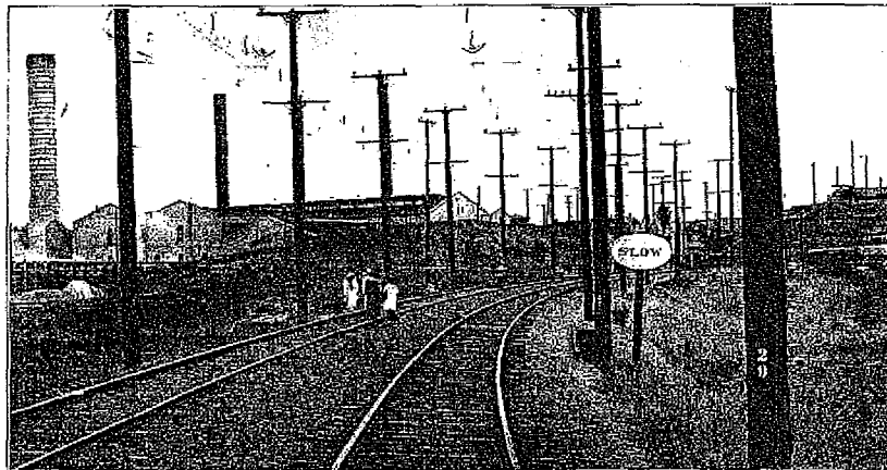
Ground view of the L approaching area at accident, show the slow board, track of rail, and trolley pole along the track.
