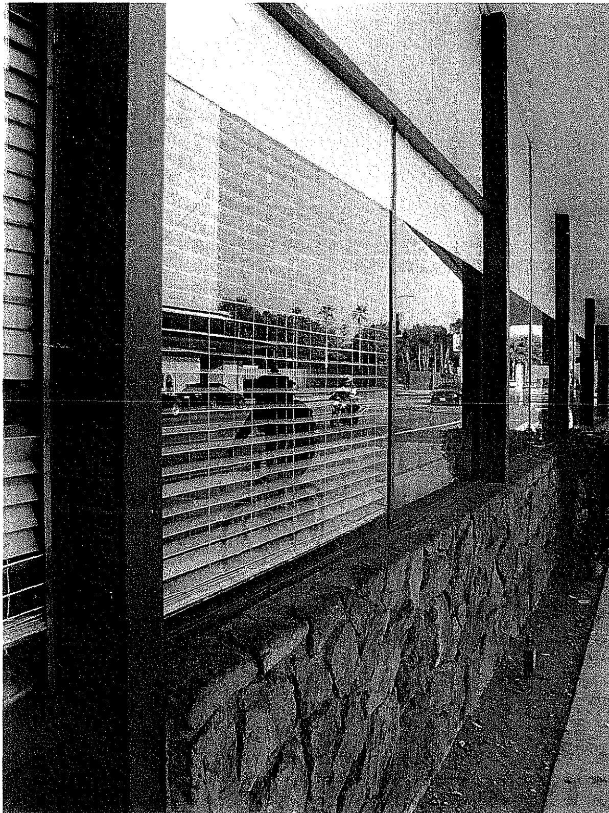
12. Johnnie's Coffee Shop Restaurant, view looking north, east elevation. (Photo by Alan Hess, 2012)
