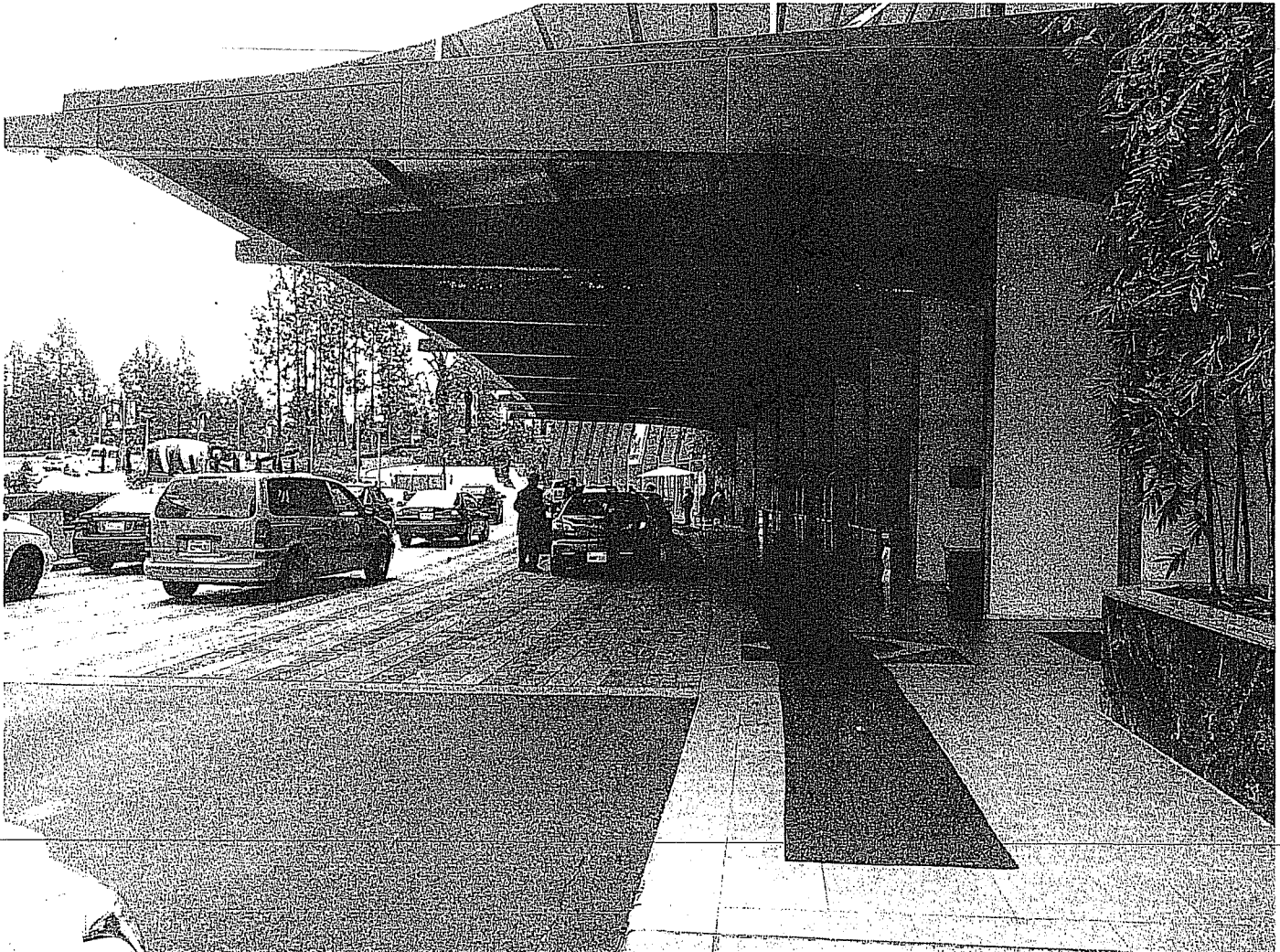
03. Detail canopy, main façade. View looking south
