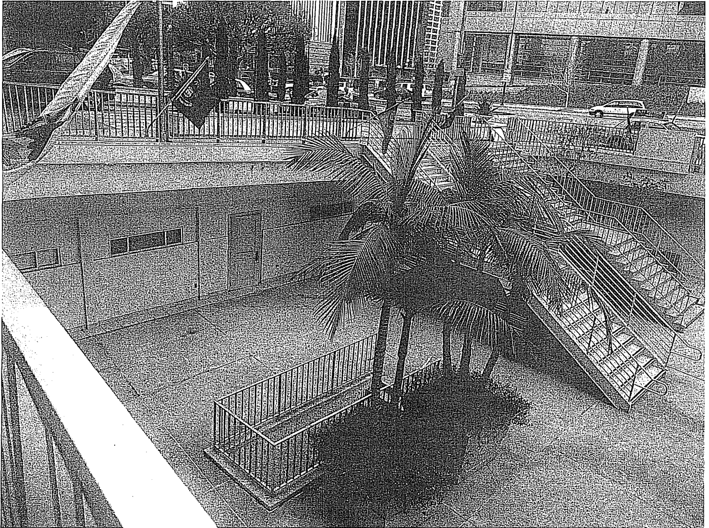
14. Sunken plaza, south-facing elevation
