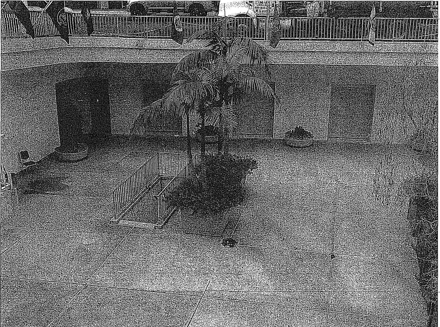
09. Sunken plaza, east-facing elevation
