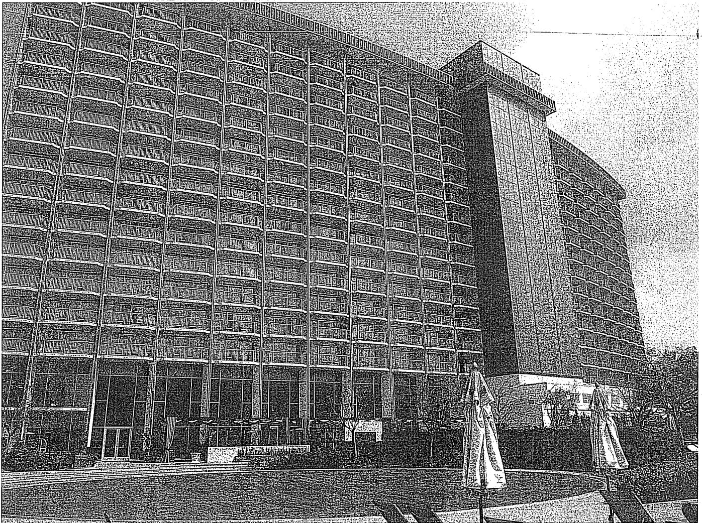
16. West façade, view looking southeast
