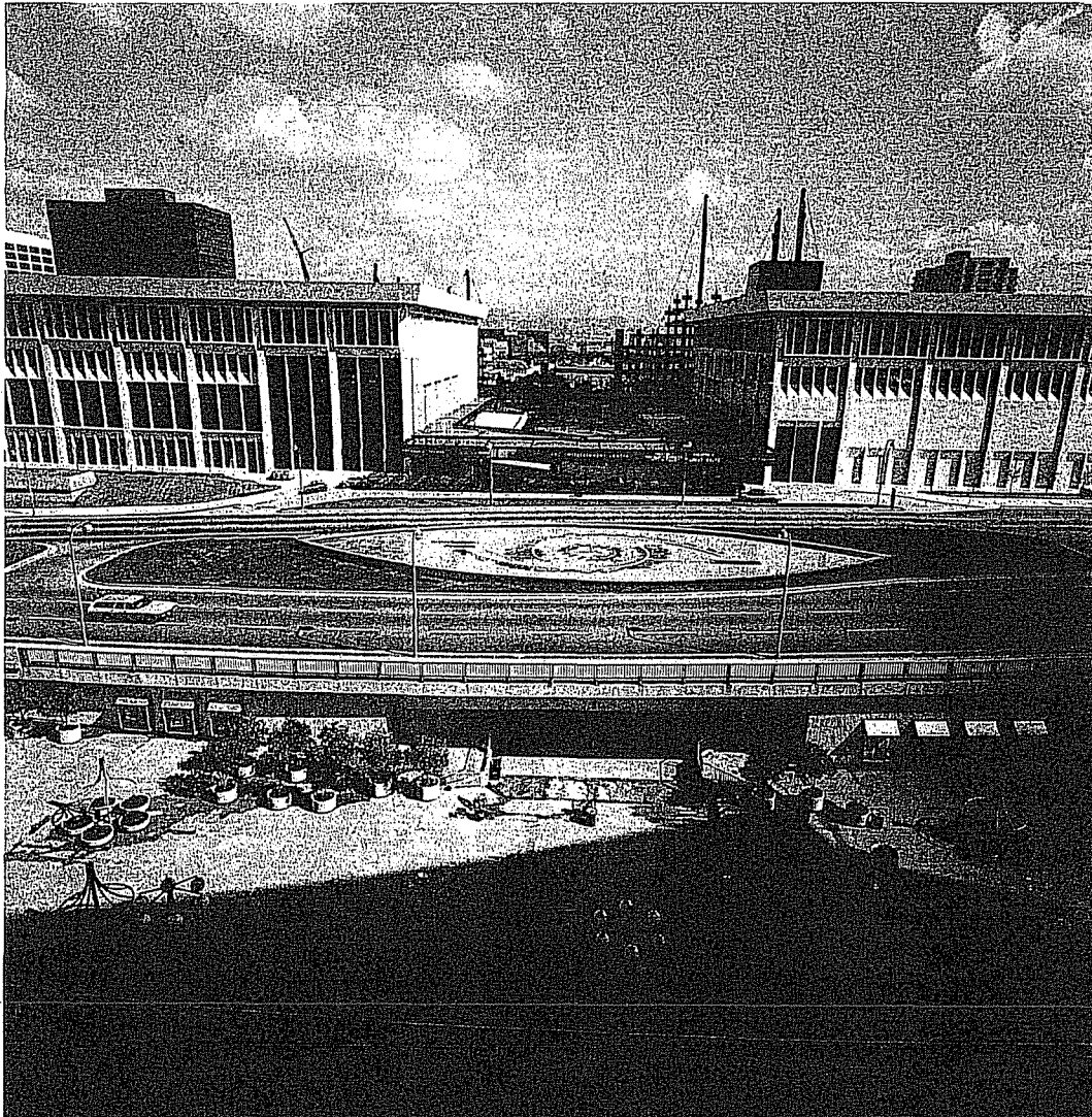
View from guest room of overall axial arrangement of site with plaza and pedestrian underpass/tunnel in foreground, c. 1960s. (Source: Courtesy Westin Hotels & Resorts, Image No. 656b280f36_1.11.)
