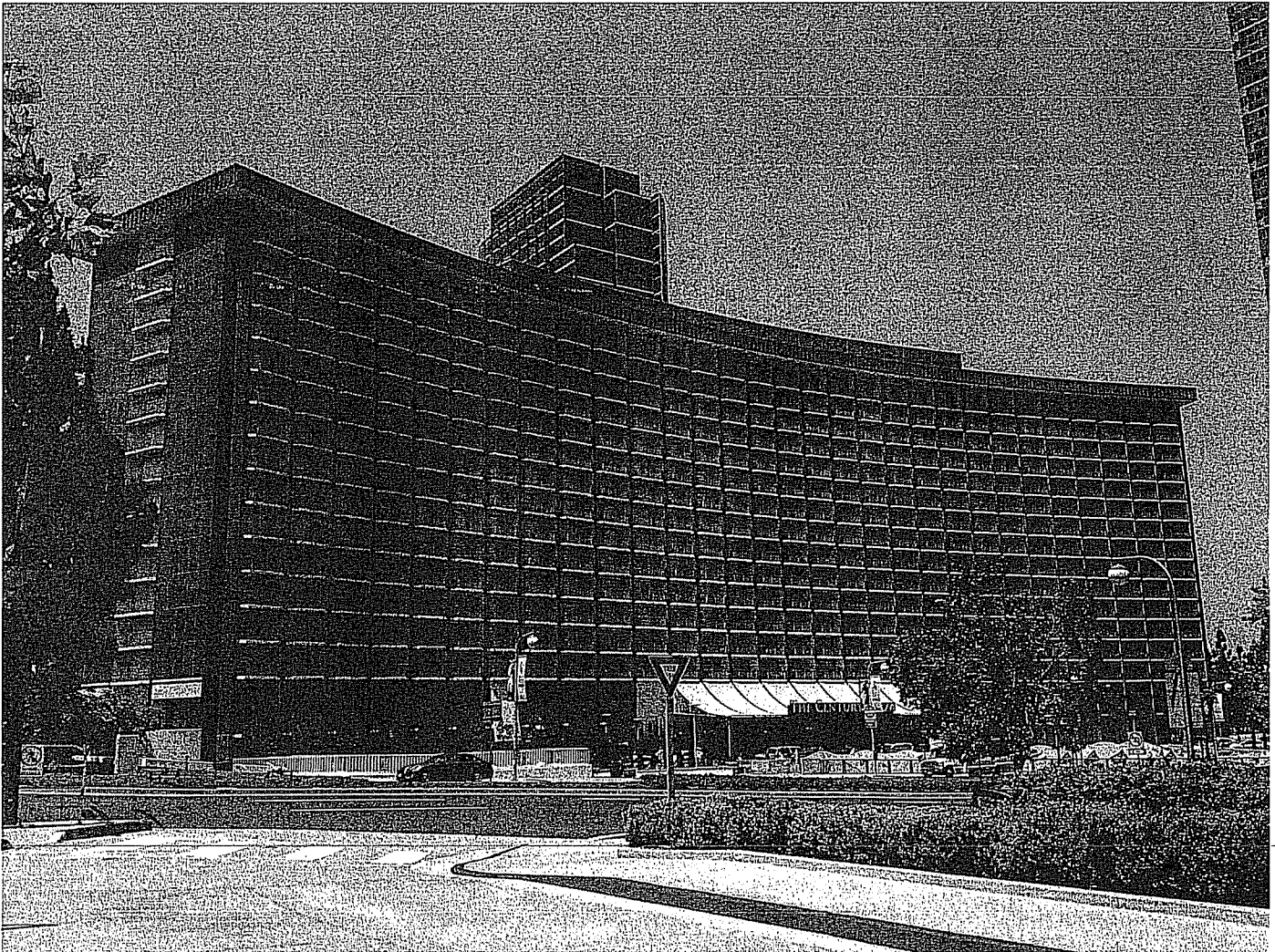
01. Main (east) façade, view looking northwest
