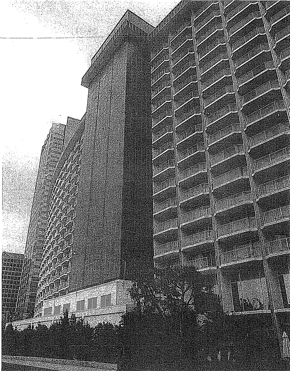
18. West façade detail, view looking northeast
