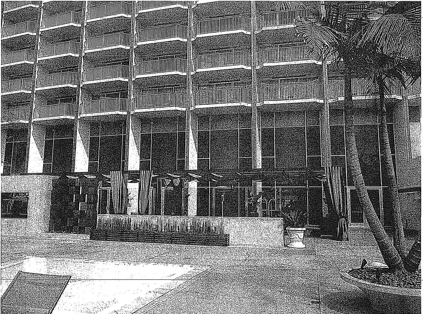
19. West façade and pool detail
