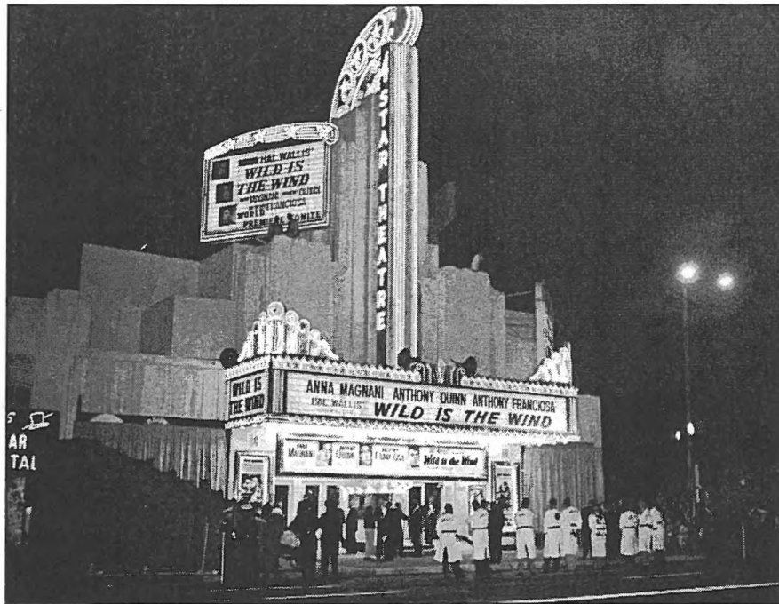
Figure 45: North façade, view southwest (Bison Archives, 1957)
