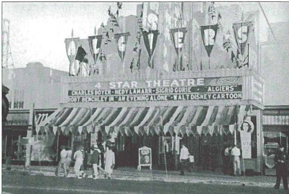
Figure 36: North façade, premier of "Algiers," view southeast (Los Angeles Public Library, 1938)
