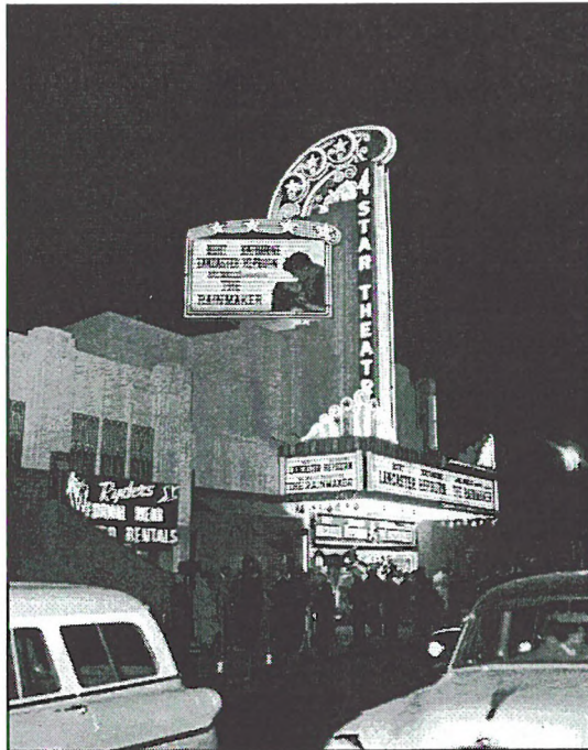
Figure 43: North façade, view southwest (Bison Archives, 1956)
