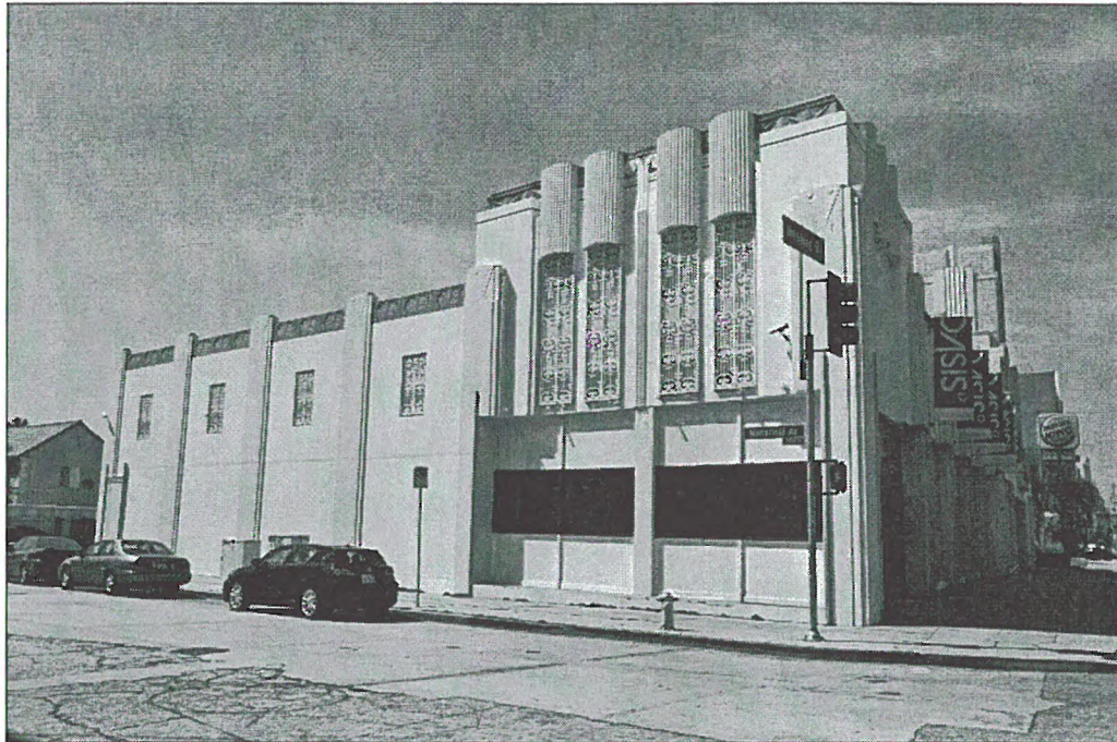
Figure 5: East elevation, view southwest (Chattel, 2013)
