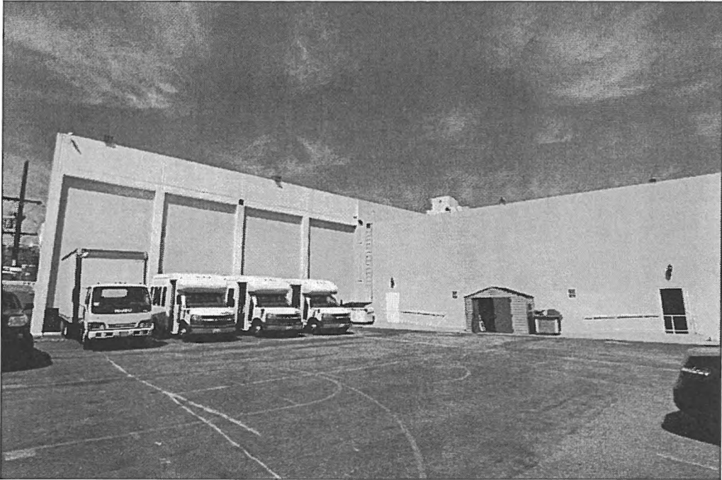
Figure 7: South elevation (right) and east elevation (left), view northwest (Chattel, 2013)
