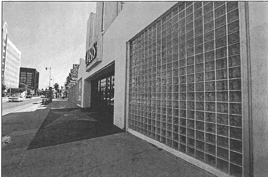
Figure 4: North elevation, main entrance, view east (Chattel, 2013)
