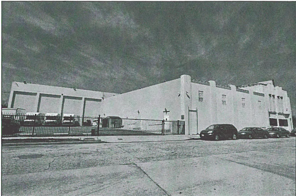
Figure 6: East elevation, view west (Chattel, 2013)
