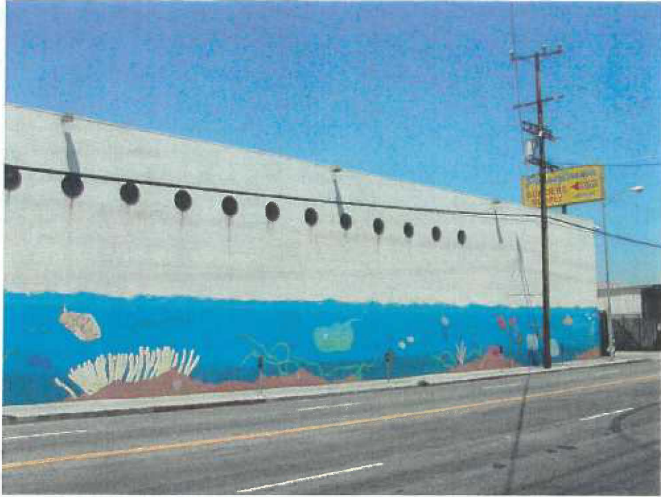
19. View looking northeast of southern edge of site from across Santa Monica Blvd.
