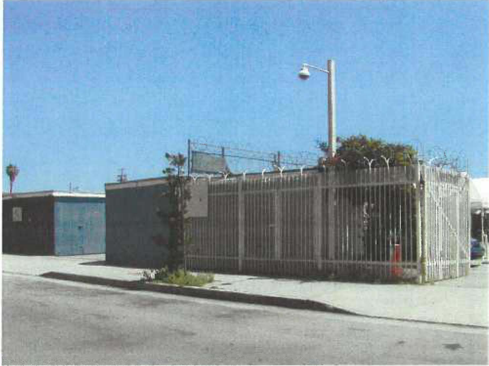
21. View looking southeast of northern edge of site from across Lexington Ave.
