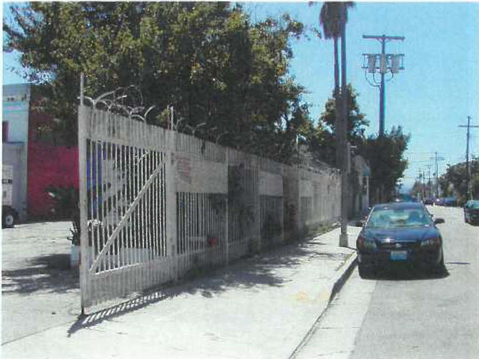
24. View looking southwest of northern edge of site on Lexington Ave.
