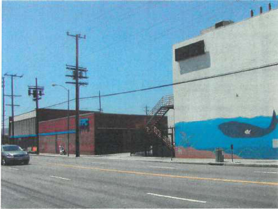
11. View looking northwest at southwestern portion of site from across Santa Monica Blvd.
