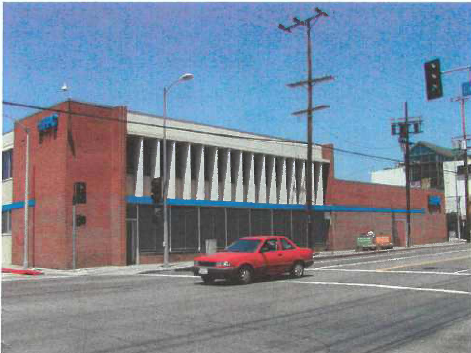
10. View looking northeast at southwest portion of site from across intersection at Santa Monica Blvd & Las Palmas Ave.
