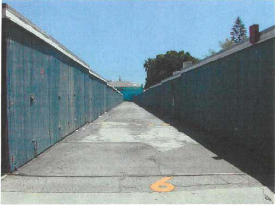
25. View looking south down typical driveway of storage site from Lexington Ave.
