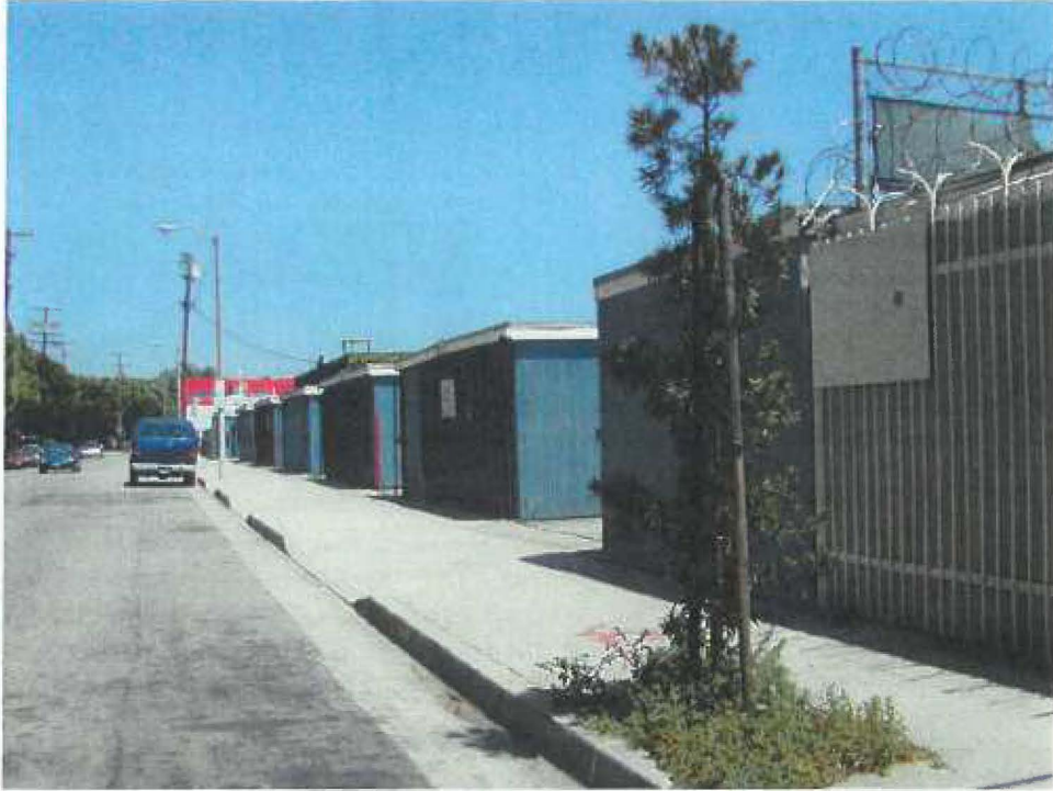
23. View looking southeast of northern edge of site on Lexington Ave.
