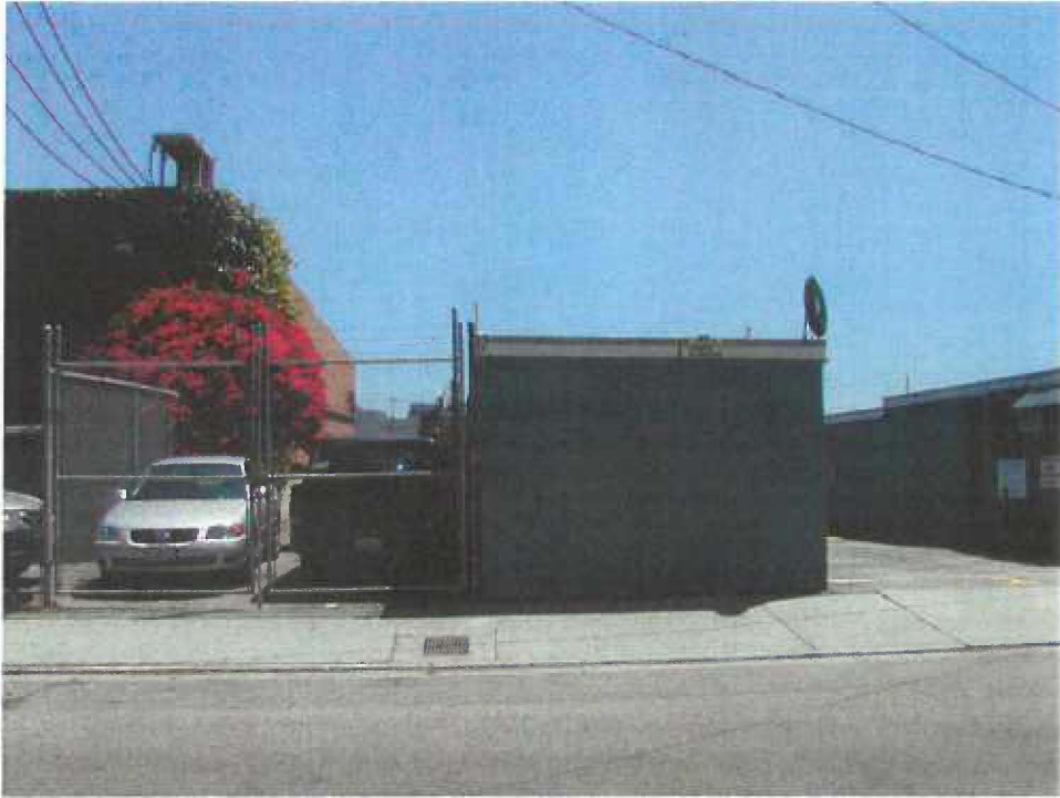
29. View looking south at eastern edge of site from across Lexington Ave.
