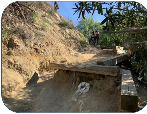
Figure 20. Erosion on Inspiration Point Trail Stairs
