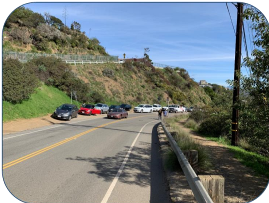
Figure 16. Unpaved Parking Along Mulholland Drive
