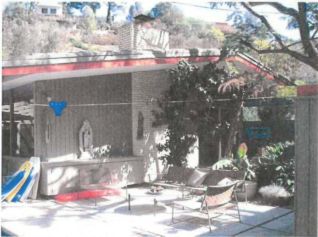
Zeiger House, 8941 Wonderland Park Avenue, South facade, October 21, 2013 (Photograph by Charles J. Fisher)
