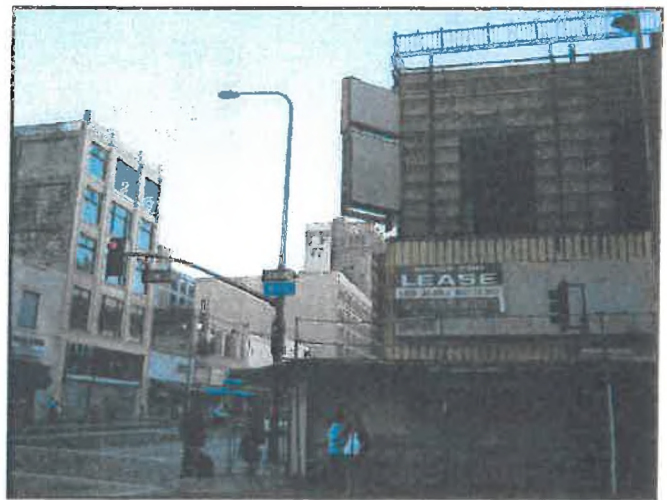
View 6: View northeast across 4th Street toward commercial/retail uses (under renovation).
