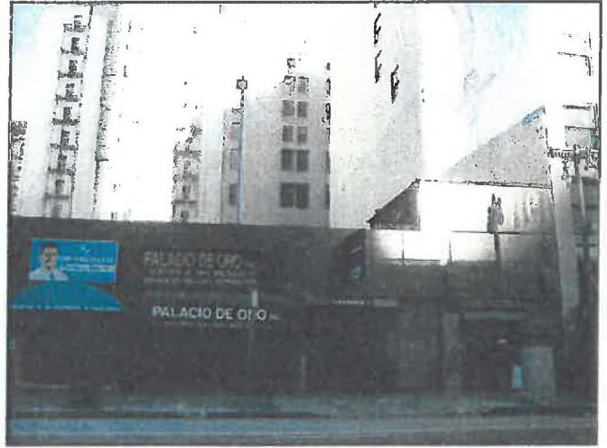
View 18: View east across Broadway toward Project Site existing building.
