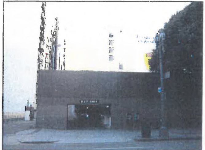
View 24: View south across 4th Street toward Project Site existing building and parking entrance.
