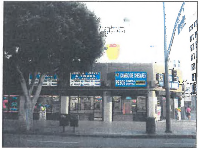
View 22: View south across 4th Street toward Project Site existing building.
