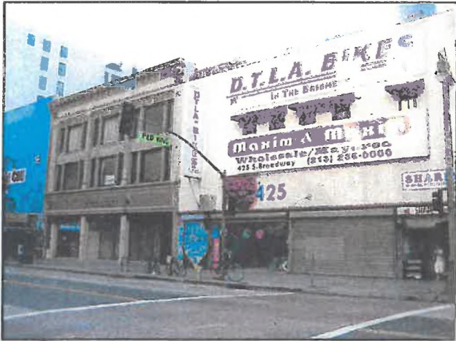
View 15: View southwest across Broadway toward commercial/retail buildings.
