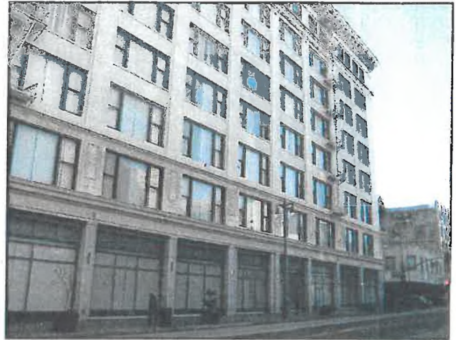
View 14: View northwest across Broadway toward Junipero Serra Office Building.
