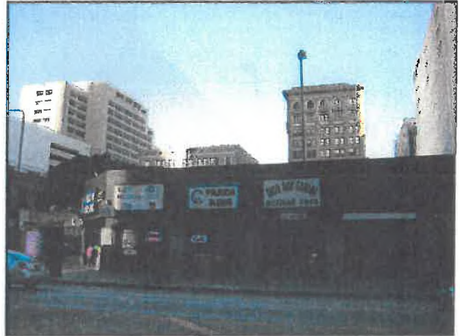
View 20: View east across Broadway toward Project Site existing building.
