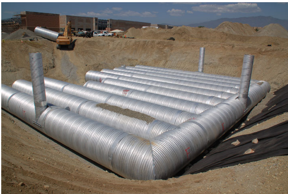
Figure 4 Photograph Storage/Detention System Using CMP (Contech, 2015)
