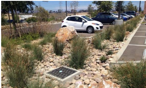
Recently constructed biofiltration in a parking lot
