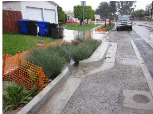
Example of bioretention and permeable pavement retrofits during construction, San Diego, CA
