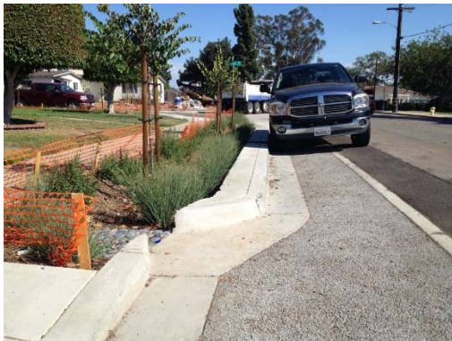
Typical residential green street
