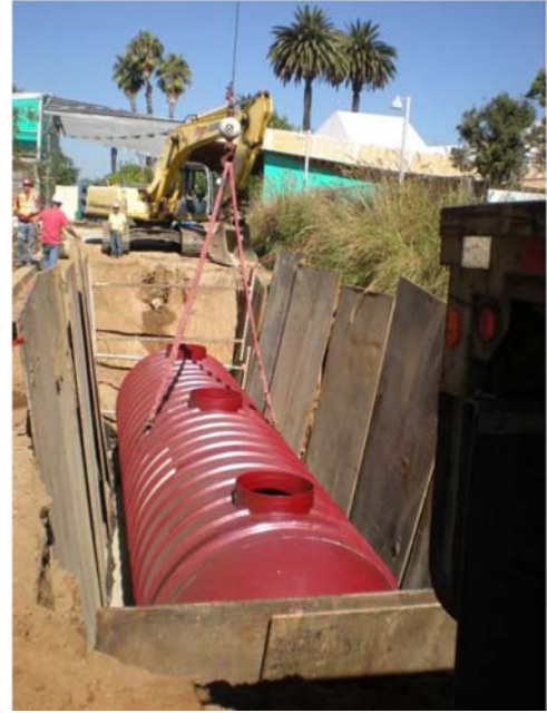
A subsurface storage tank and treatment system being installed (source: Neal Shapiro, City of Santa Monica)
