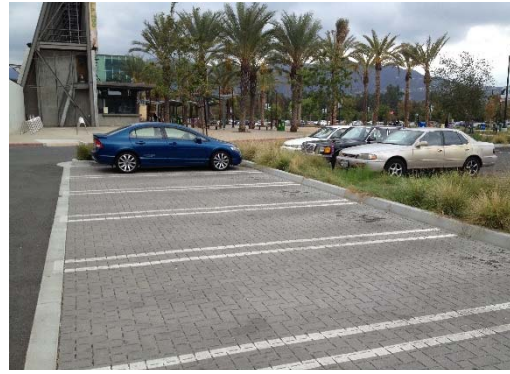
Bioretention and permeable pavement at the Los Angeles Zoological Park
