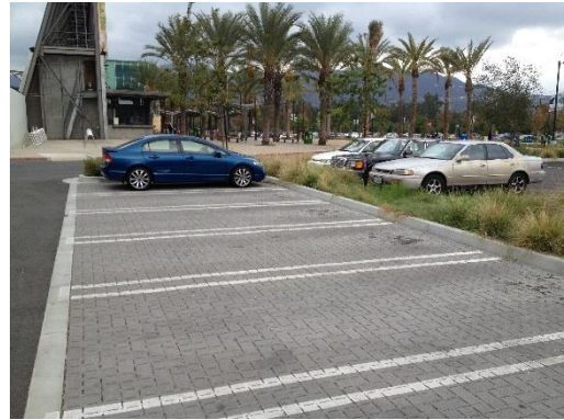
Figure 5-9 Bioretention and Permeable Pavement at the Los Angeles Zoological Park
