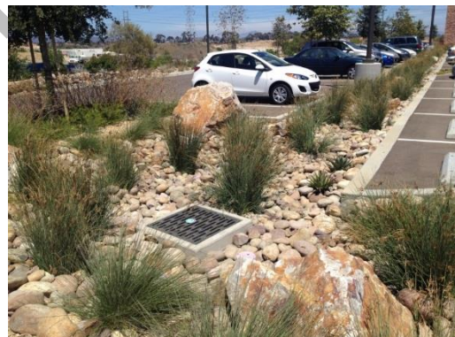
Figure 5-10 Recently Constructed Biofiltration in a Parking Lot
