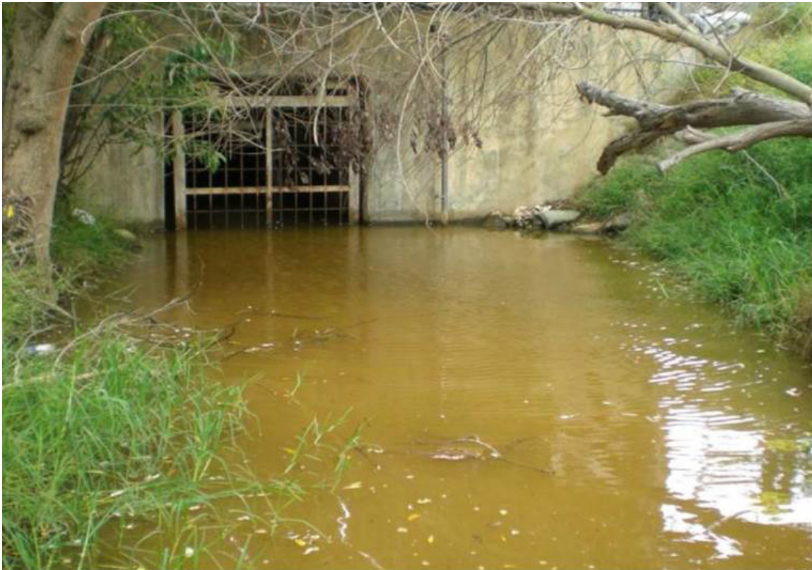
Drainage at Marie Canyon Low-Flow Diversion.
