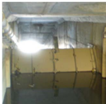
Marie Canyon Low-Flow Diversion – Flat Gate Diverting flow to treatment unit for bacteria
