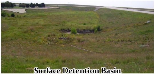
Surface Detention Basin
