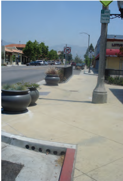
Large sidewalks with curb bulb-outs encourage businesses to provide landscaping and orient their entrances towards the public street create a more inviting streetscape to pedestrians and customers.
