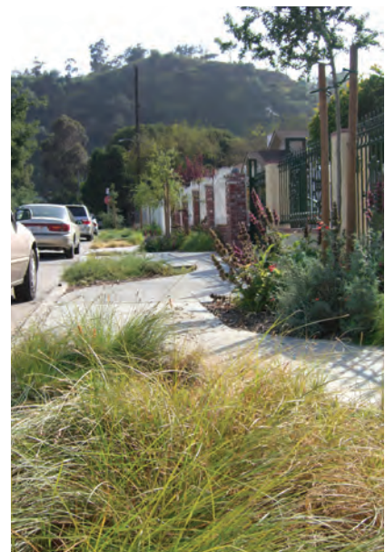
Bioswales in the streetscape design of a neighborhood can increase storm water infiltration and remove pollution and silt from surface runoff water.
