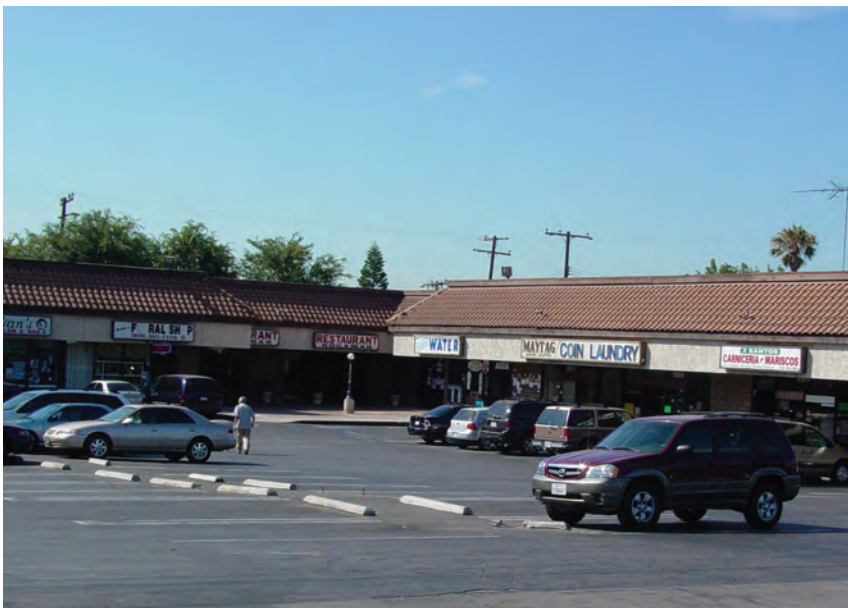
Existing condition of commercial center with a mix of uses.
