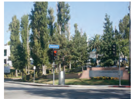
The North Valley Business Center, located on Telfair Avenue, is one of the main industrial parks within the community of Sylmar, providing employment opportunities.
