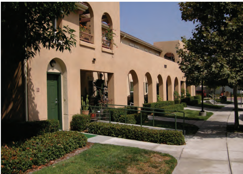
Architectural features such as arches, articulation and patios, combined with landscaping can help enhance the appearance of multiple family housing, as well as maintain small scale neighborhood settings.
