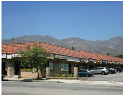
Typical single-story commercial development in Sylmar.
