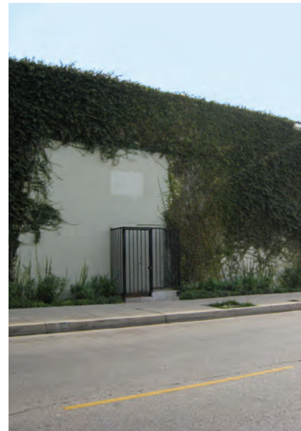
An industrial building with wall-climbing vines.
