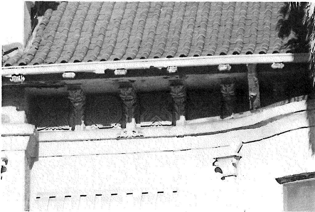
Details: Gutter brackets, eaves with decorative brackets with decorative plaques between them. Decorative member on banding. Decorative members on downspout headers.
