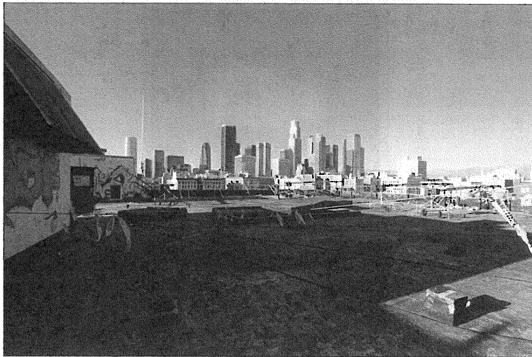
Photo 10: Maxfield Building, 819 S. Santee Street, exterior view west of roof, during current adaptive reuse project (Chattel, 2014)
