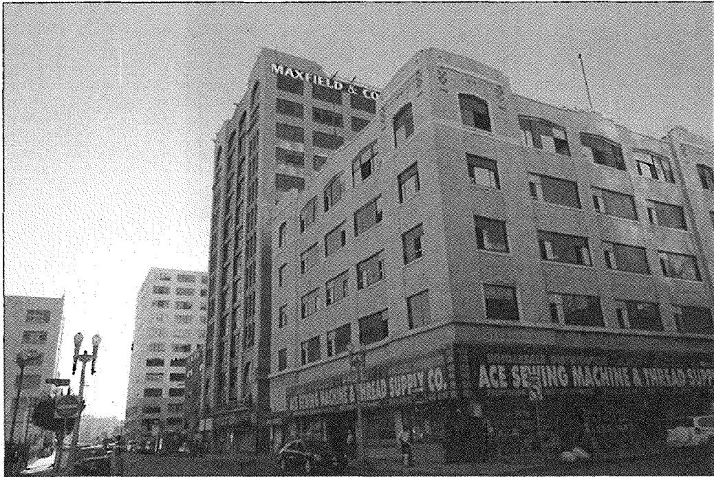
Photo 5: Maxfield Building, 819 S. Santee Street, exterior view southwest of east façade and north elevation, during current adaptive reuse project (Chattel, 2014)
