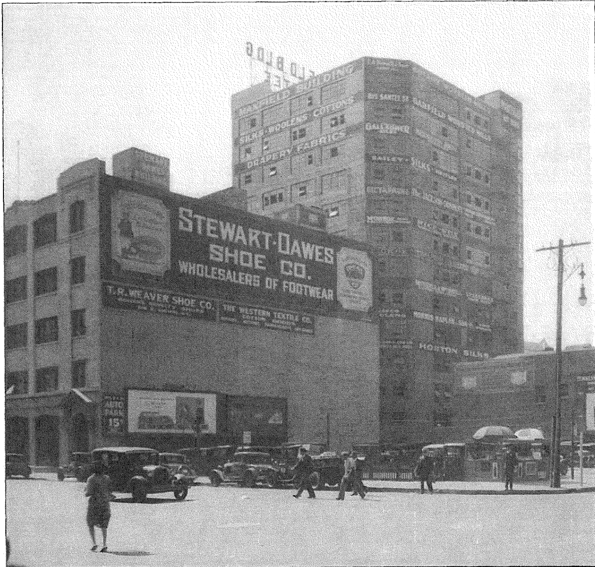
Figure 11: Maxfield Building (at center), north and west elevations, (USC Libraries Special Collections, 1931)
