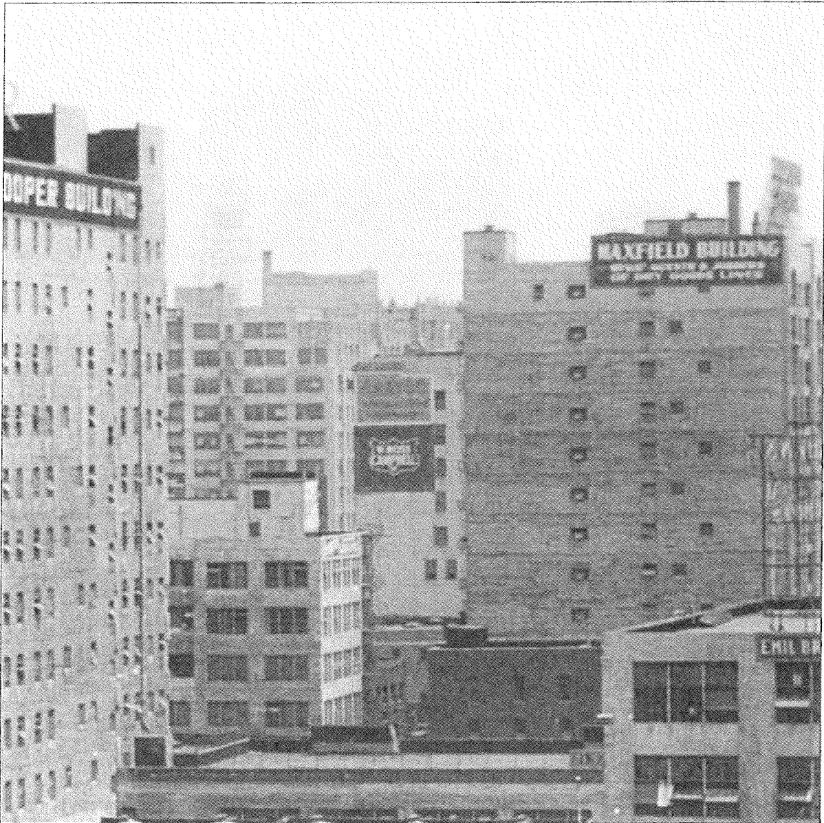
Figure 10: Maxfield Building (right), south elevation (USC Libraries Special Collections, 1927)
