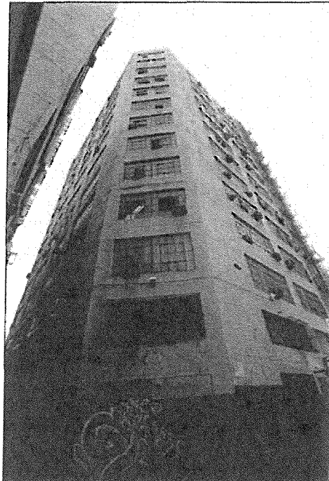
Photo 4: Maxfield Building, 819 S. Santee Street, exterior view southeast of north and west elevations (Chattel, Inc., December 4, 2012)
