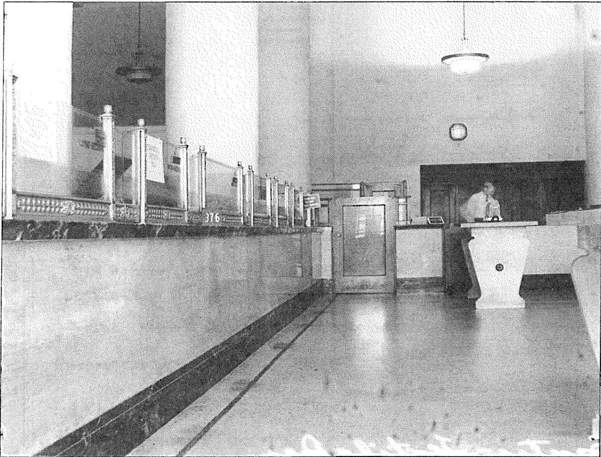
Figure 22: Interior of Bank of America Santee-Textile branch at Maxfield Building (Bank of America Historical Collection, 1940-1941)
