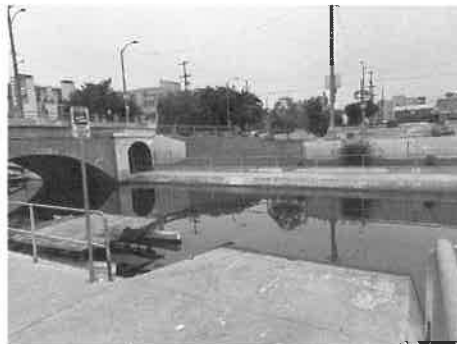
VENICE CANAL BOAT LAUNCH RAMP
