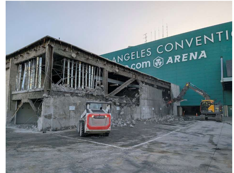
Existing arena conditions informing DD-level signage coordination and procurement strategy.
