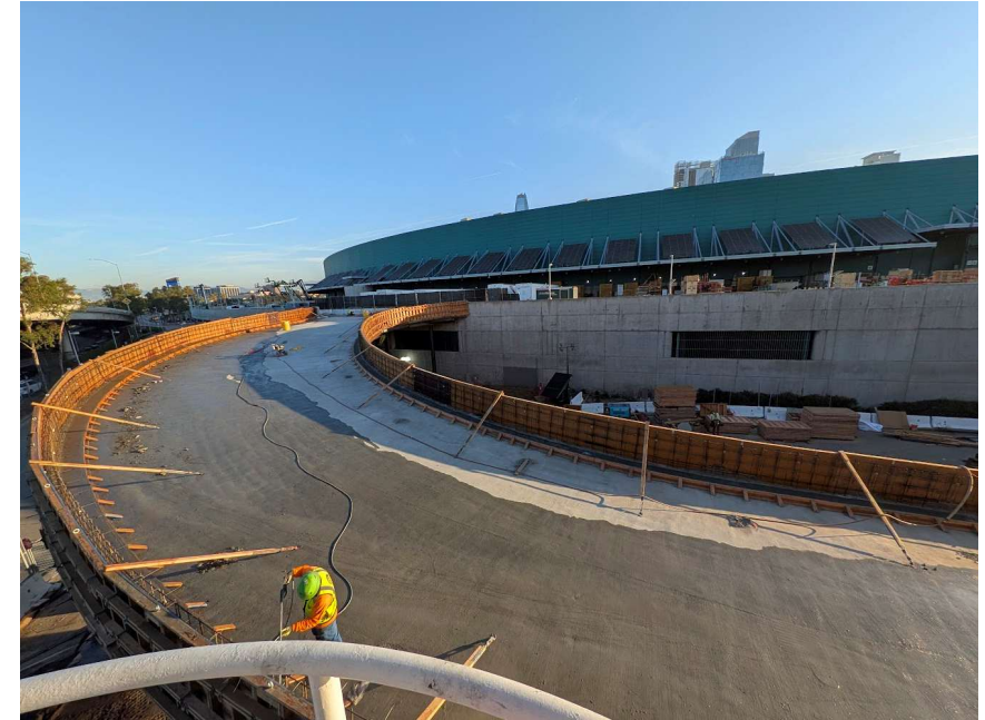
Pico Passage Pedestrian Ramp
