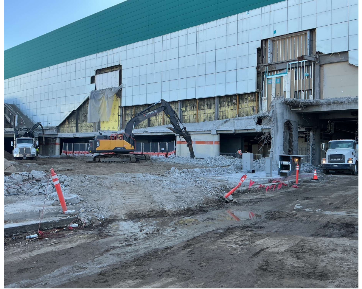
Concourse Exterior Façade Demolition – March 6, 2026
