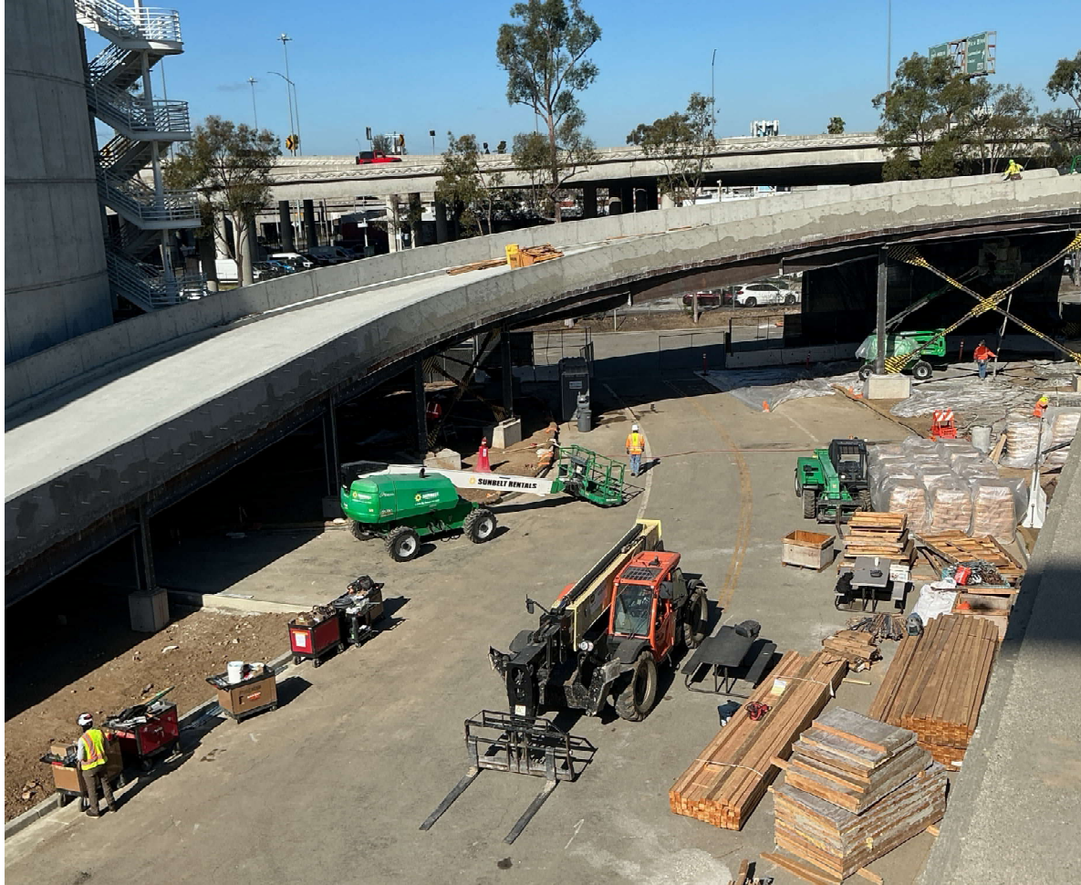
Temporary South Hall Ramp – March 6, 2026
