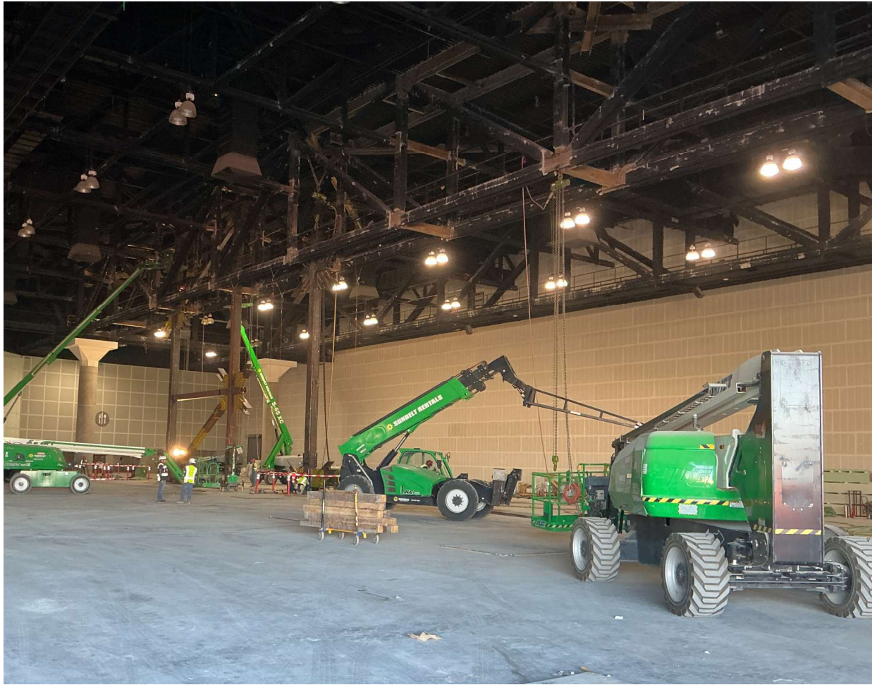
South Hall Truss – March 6, 2026
