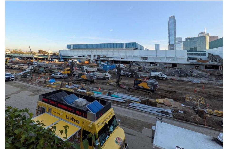
Site conditions supporting Early Foundations and critical permitting progress.
