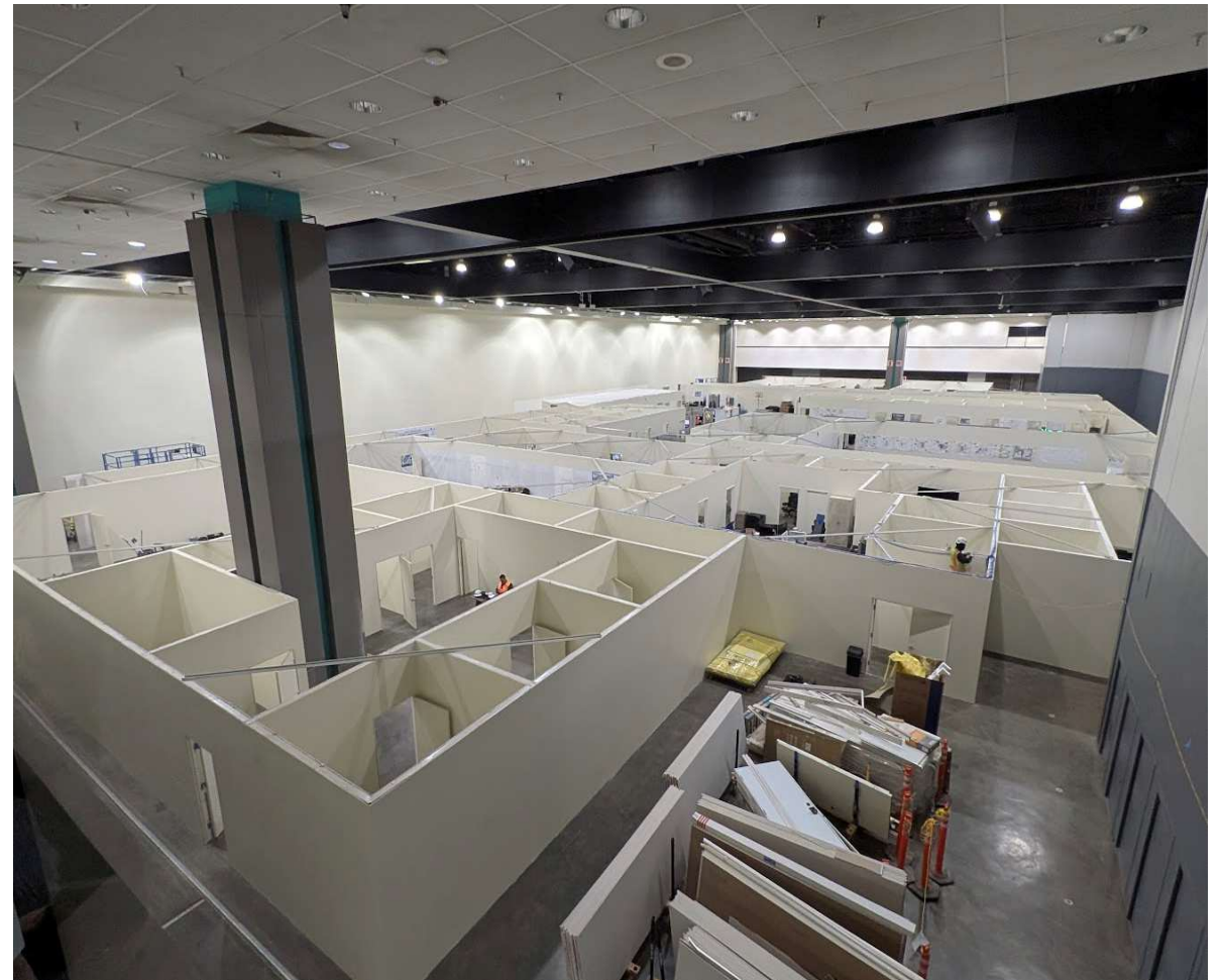
Build Out of Staff Offices at Convention Center
