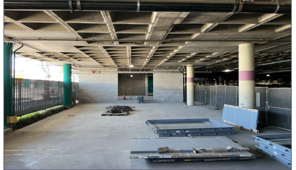
Continuing work on new Fire Command Center room underneath West Hall
