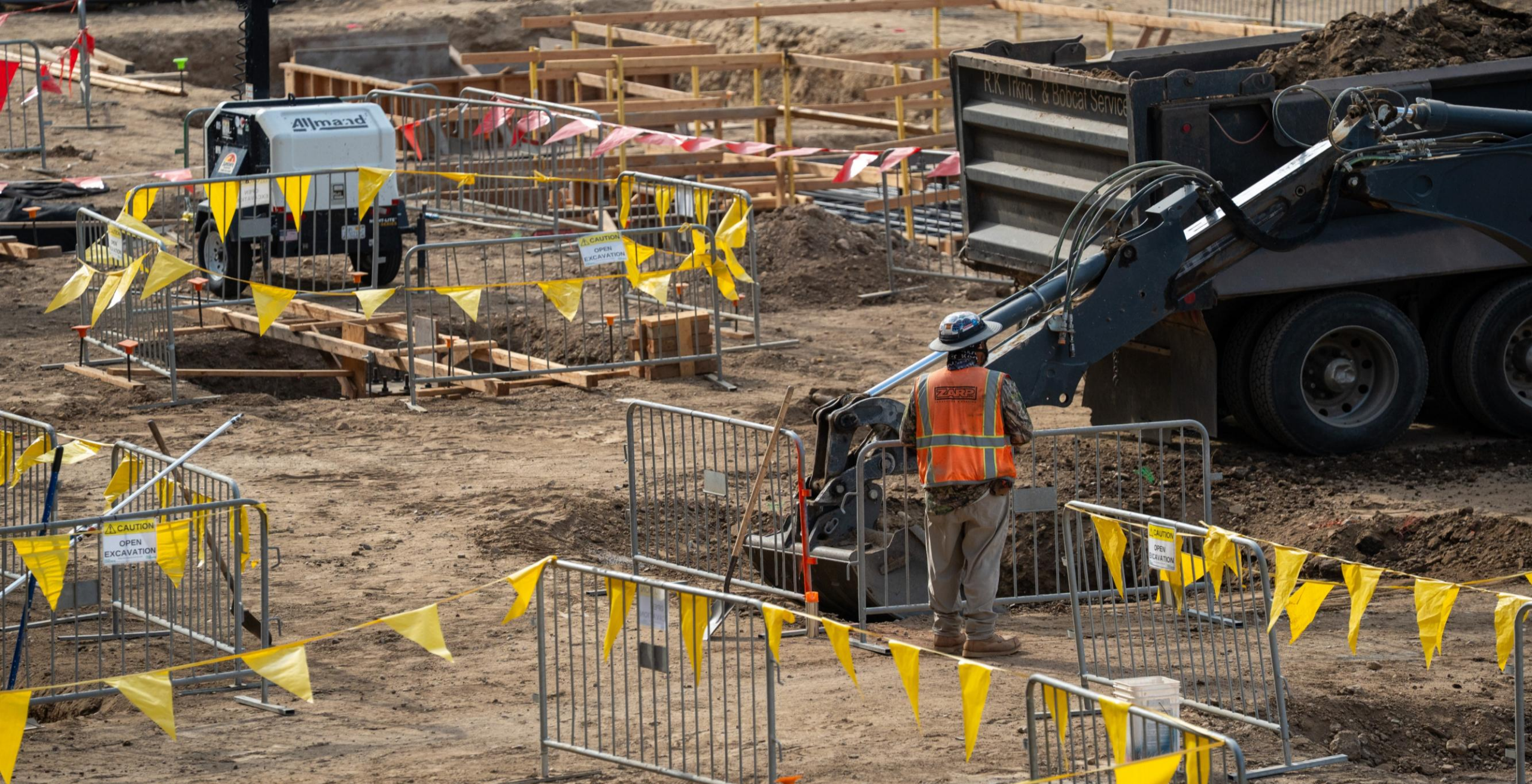
Foundation excavation and soil removal at Expansion Building site
