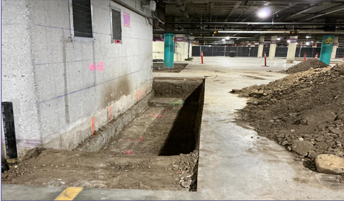
Saw-cutting to prepare for micropiles
