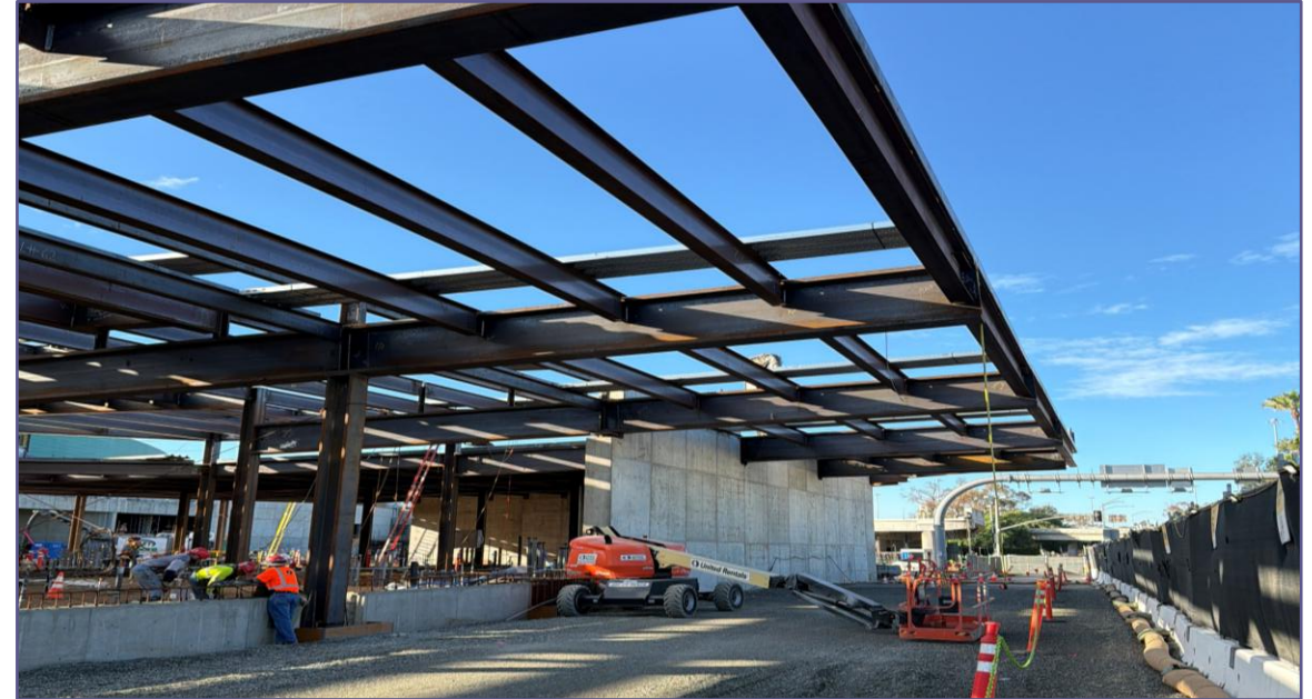
Cantilevered structural steel over LA Live Way
