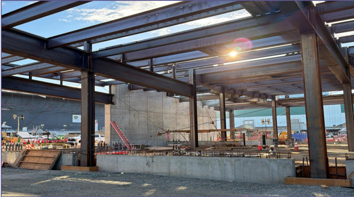
Structural steel erected within the CUP
