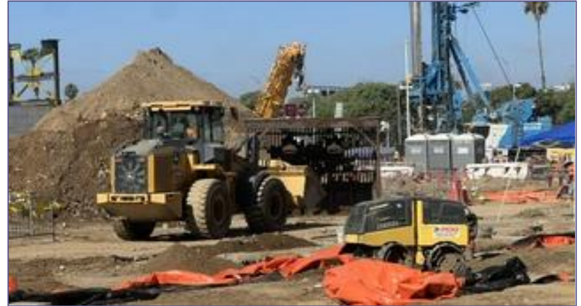
River rocks being sorted and sifted by size to prepare soil for grading and backfill
