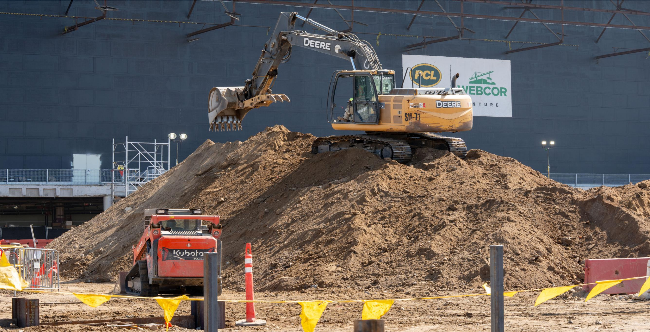
Removing excess spoil piles in order to prepare the site for foundation work
