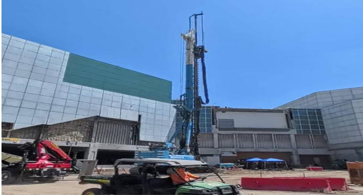
Continuation of auger cast piles
