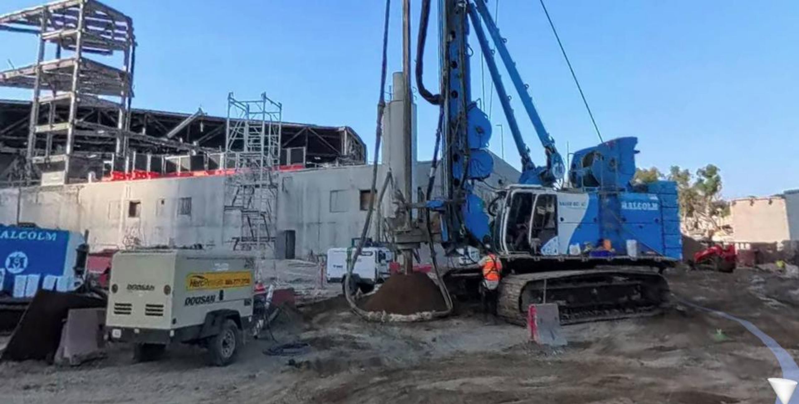
Ongoing auger cast pile being drilled near South Hall while the structural steel deck level is being dismantled.
