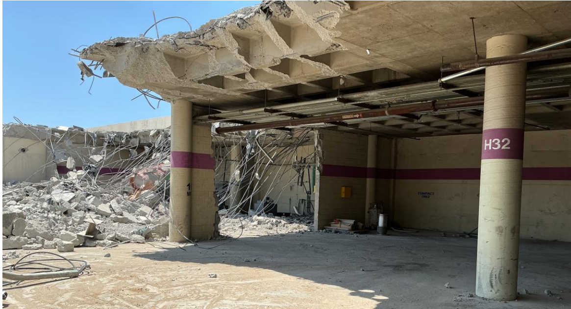
West Hall generator room demolished - temporary generators now active
