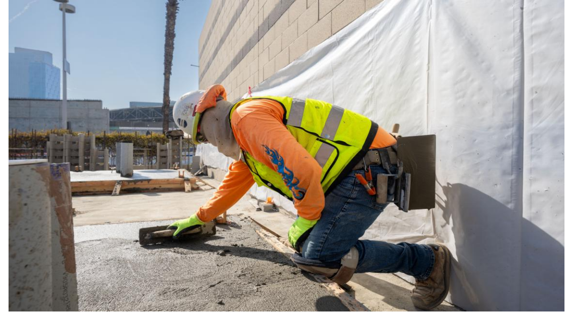
Finishing slab-on-grade foundation
