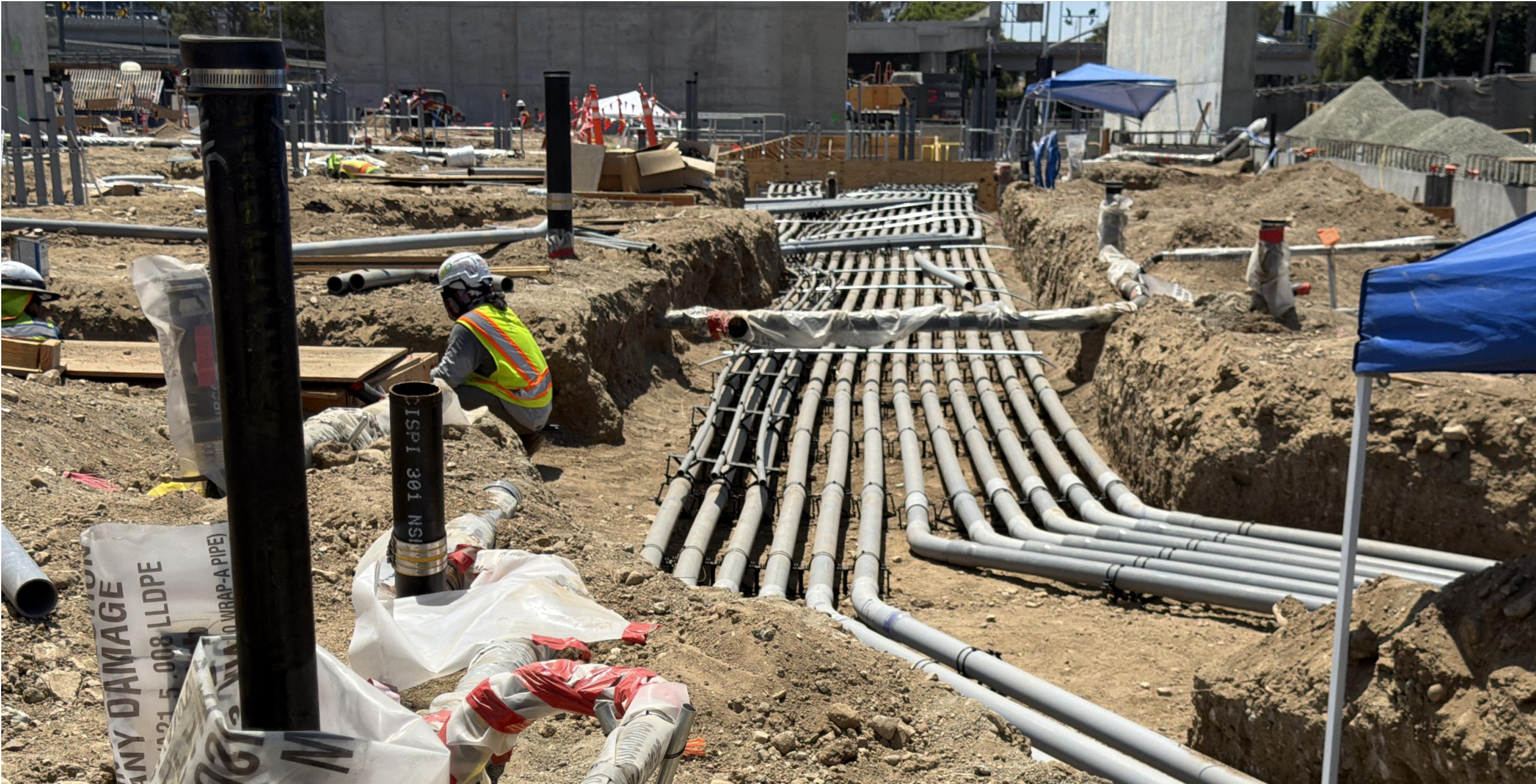
Continuing trenching and conduit installation in order to prepare site for Central Utility Plant (CUP) structural steel.
