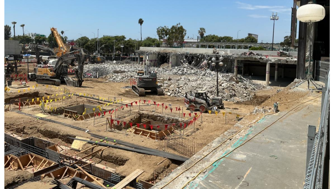
Overview of auger cast caps / foundation pours beginning
