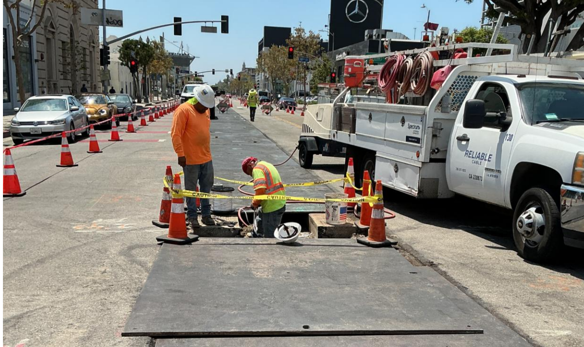
Circuit work continuing on Figueroa and Washington for expected vault placement
