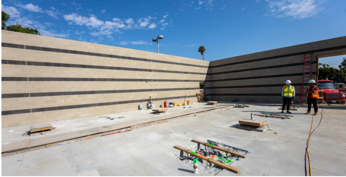
Network Station concrete masonry unit (CMU) walls erected
