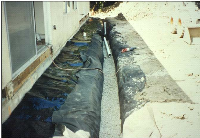
Fig.3: French drain mitigation of expansive soils
