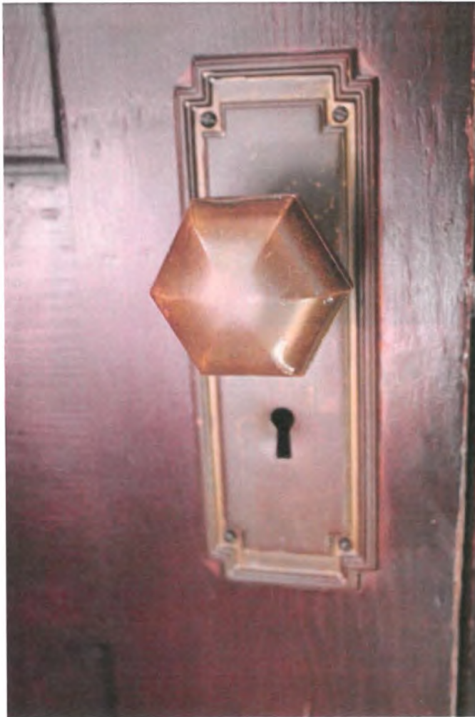
Detail: Original escutcheon & door knob used throughout.
