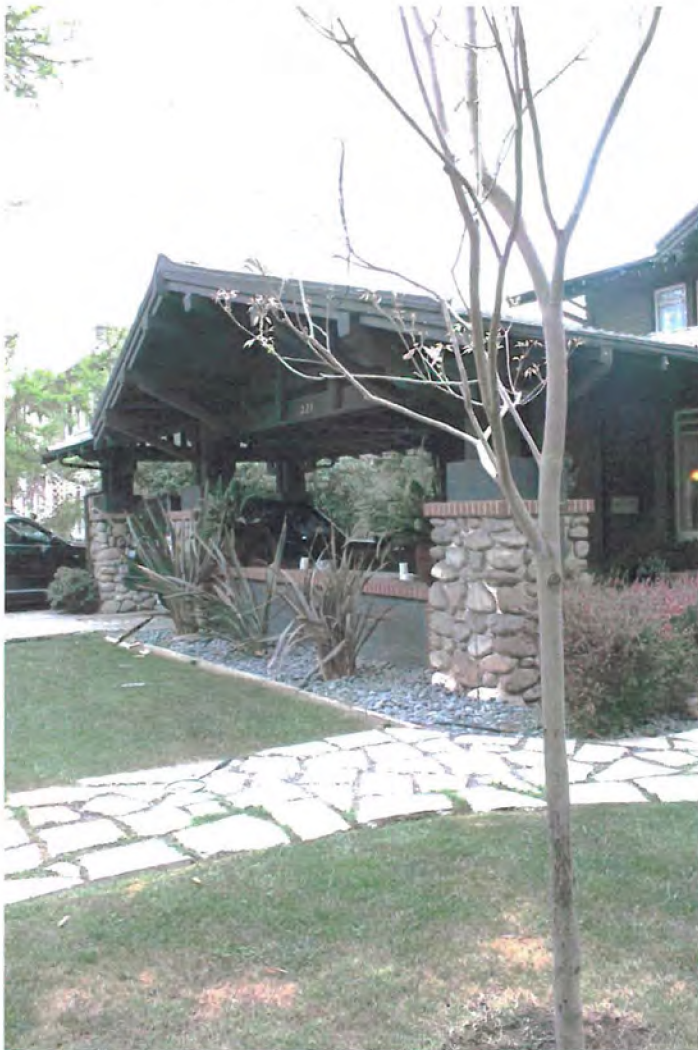
Porch of residence: View southwest.
