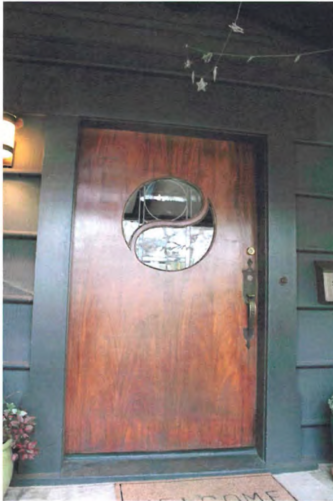
Entry door off north/south portion of raised wrapping porch; view west.
