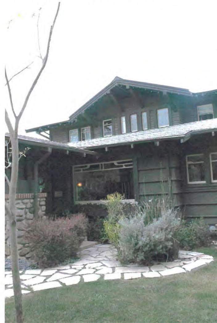
First and second story of residence with Oriental influence large single-pane window of living room: View southwest.
