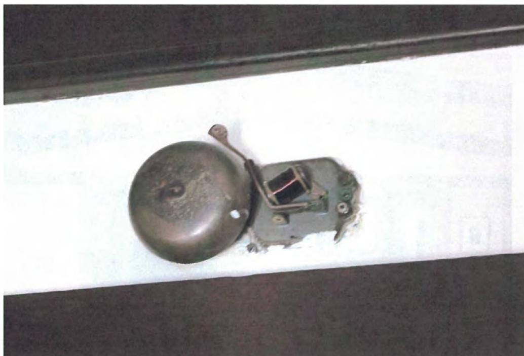
Detail: Doorbell at dining room north wall.
