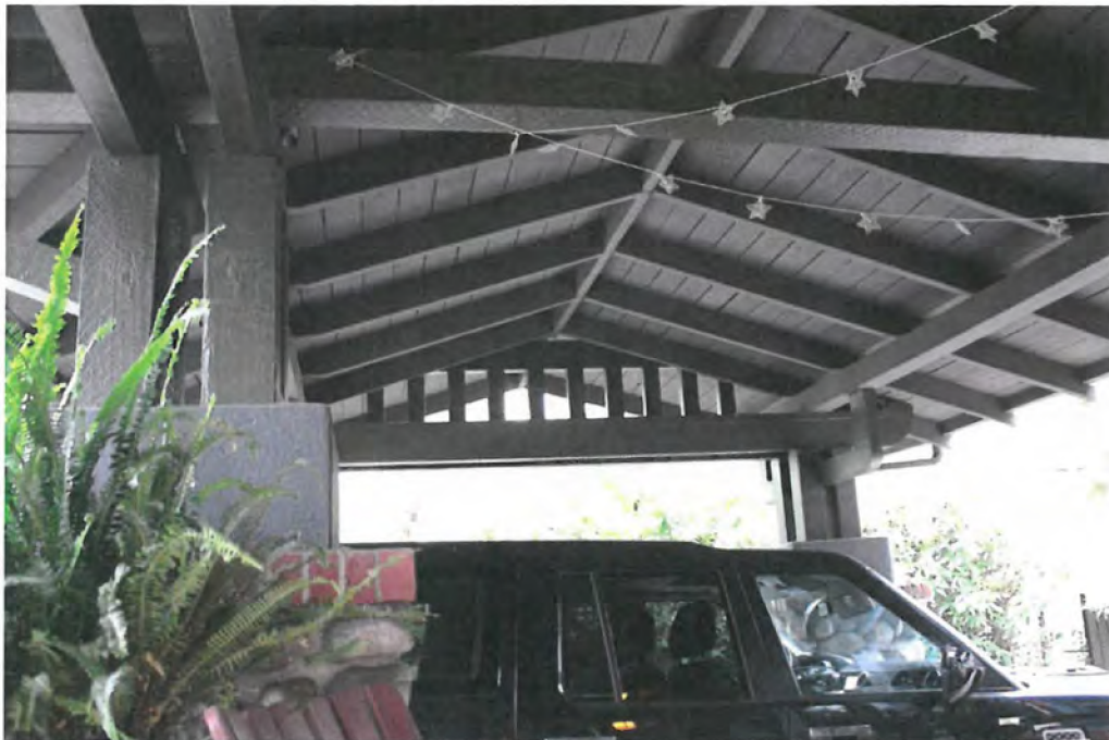
Gabled porte-cochere: Intersection of porch roof gable with porte-cochere gable above brick pier and beam upright support, view south.
