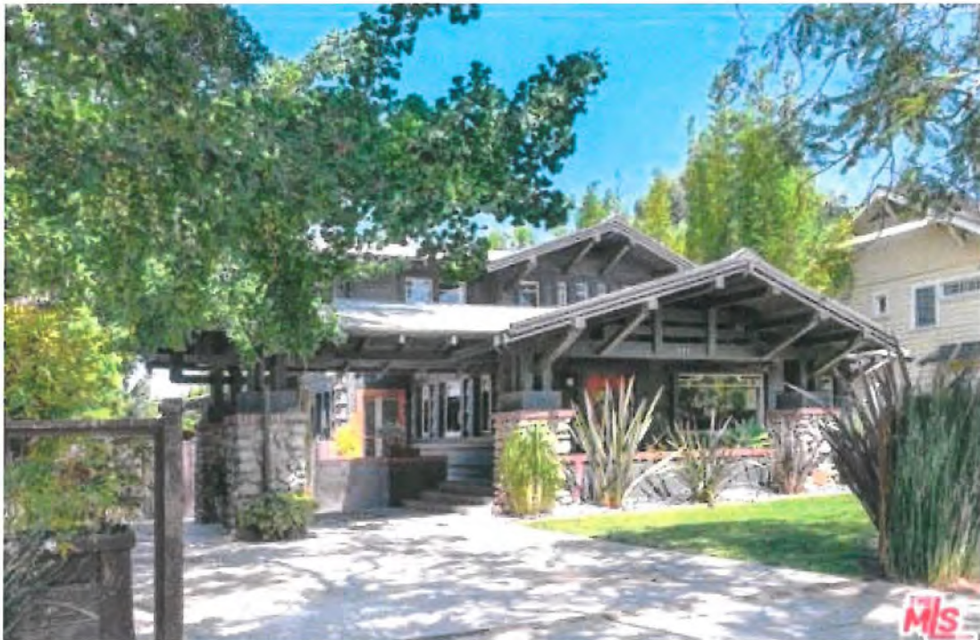
South elevation & east façade of residence, as purchased photograph from the MLS.
