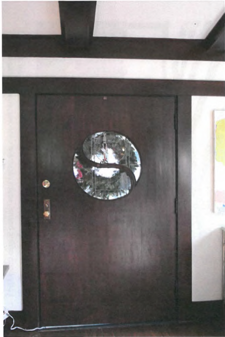
Original entry door, from interior, view east.
