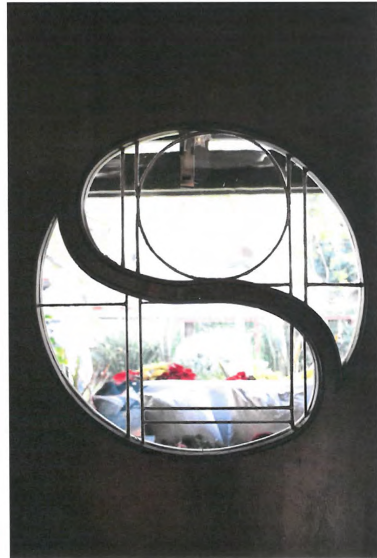
Detail: Window, original entry door, view east from interior.
