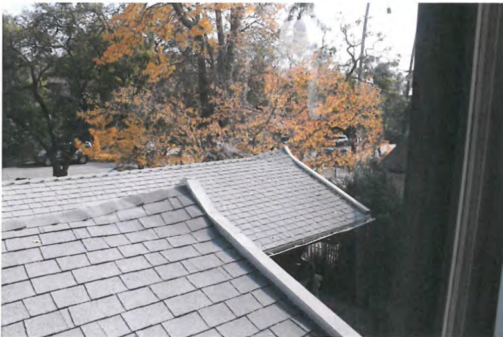
Craftsman Airplane bungalow with Oriental influence roofs: Porte-cochere and south section of porch; ginkgo tree turned golden, beyond, view southeast.
