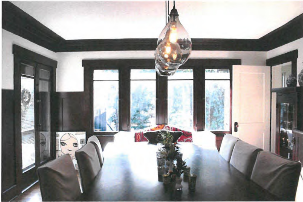
Dining room: East wall with original doors to wrap around porch; south wall ribbon of casement windows set in high paneled wainscoting; original 2-panel kitchen door and breakfast, view south.
