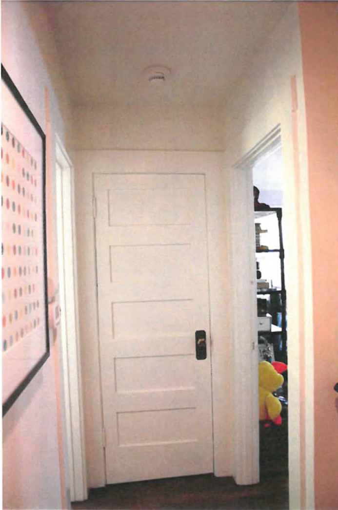
Second floor hall: View north to original 5-panel closet door.
