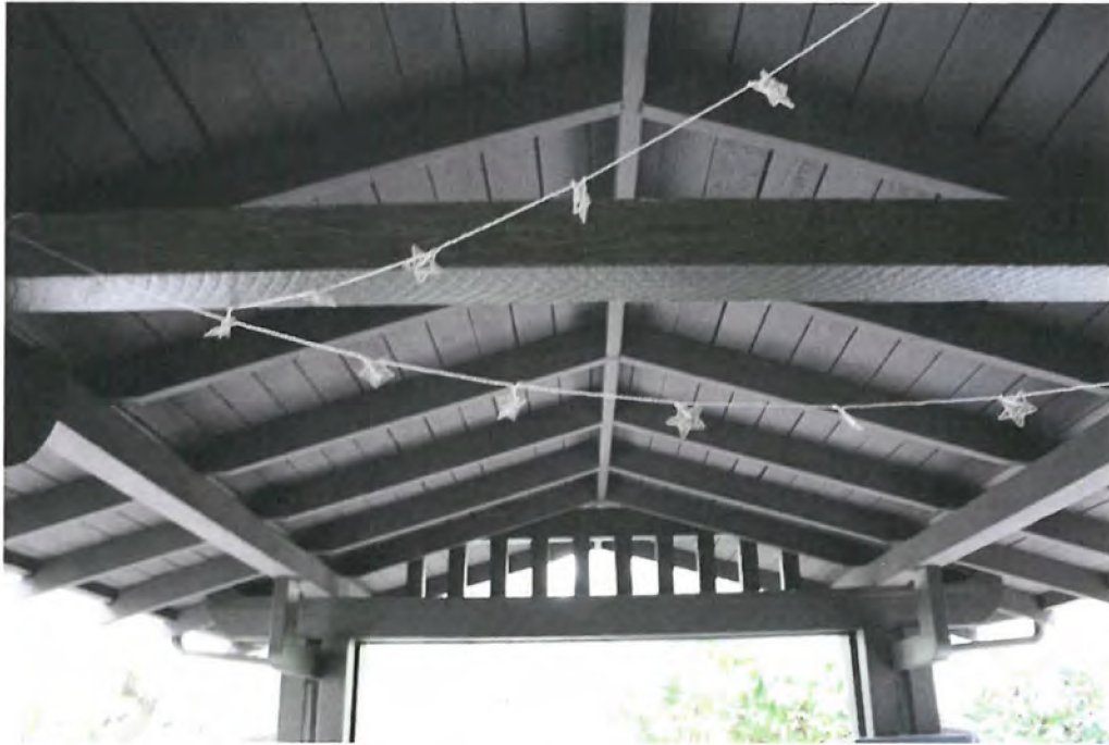
Gabled porte-cochere: South end with Oriental influence shaped beam supports and semi-open end, view south.
