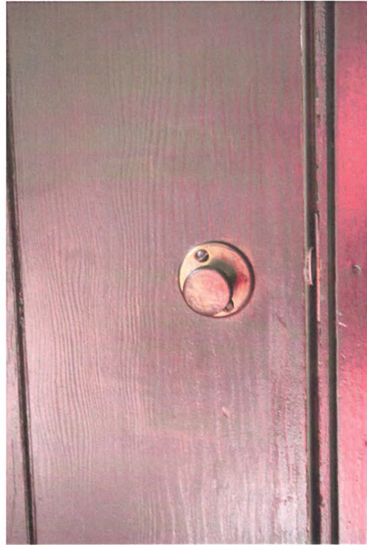
Detail: Original door locks, employed throughout.
