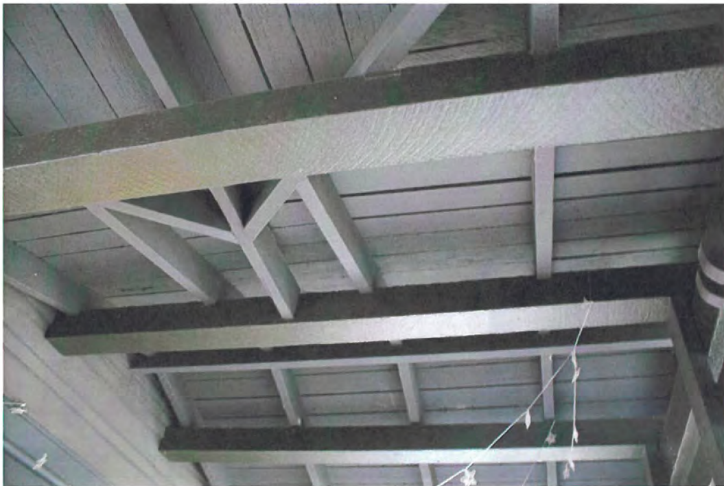
Detail: Beam work beneath porch roof.
