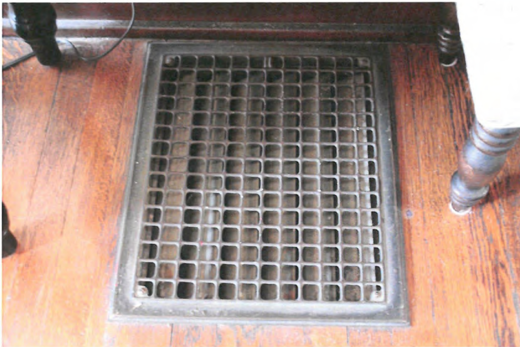
Detail: Original floor heat register.
