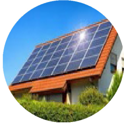
Customer Rooftop Solar
