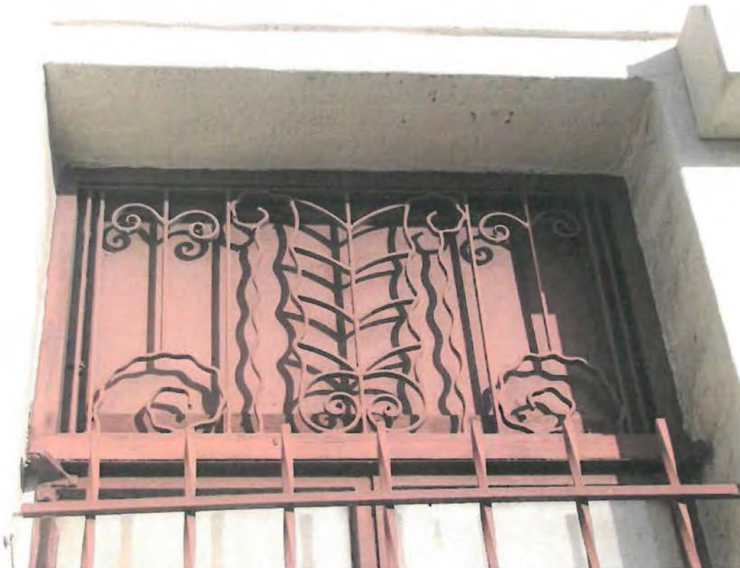
Redwine Building, window grille, 1618 N. Las Palmas Avenue, February 5, 2015 (photograph by Charles J. Fisher)
