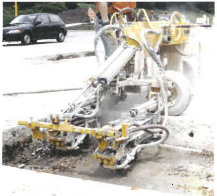
Figure 11. A gang drill, used to drill multiple dowel bar or tiebar holes simultaneously.
