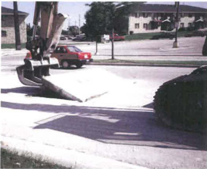
Figure 8. Partial slab removal using a clawed hook lift-out method.
