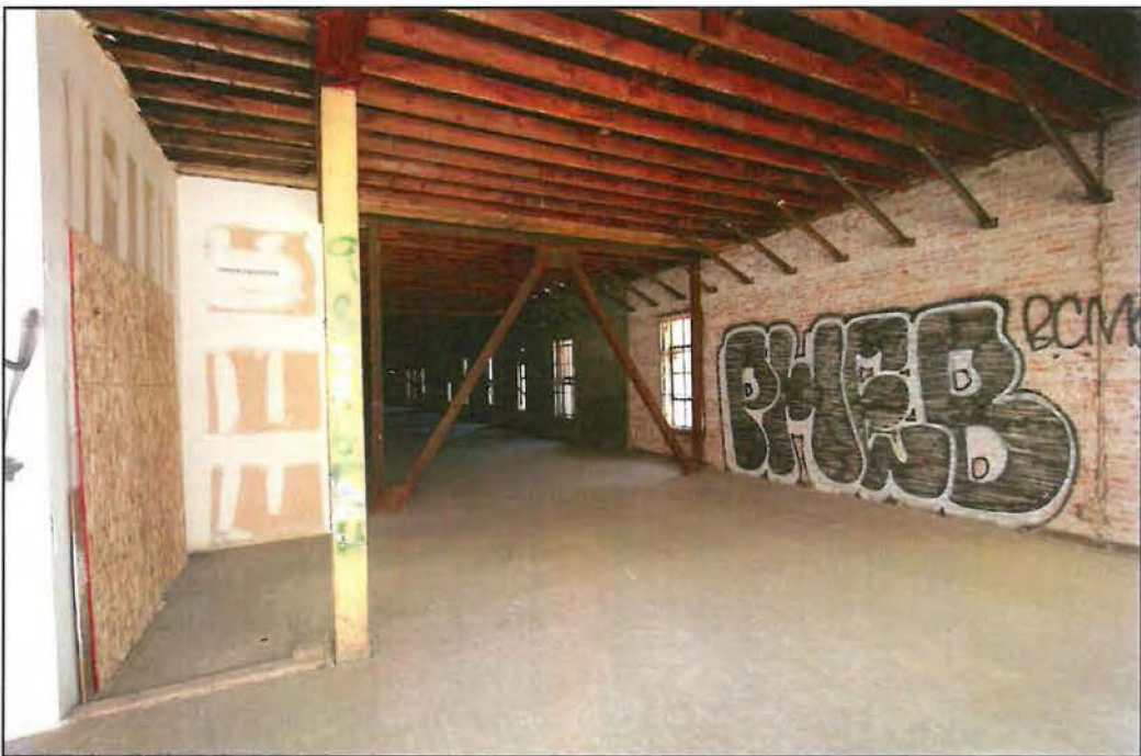
Figure 105: Interior of the fourth floor, looking east (Chattel, 2015).
