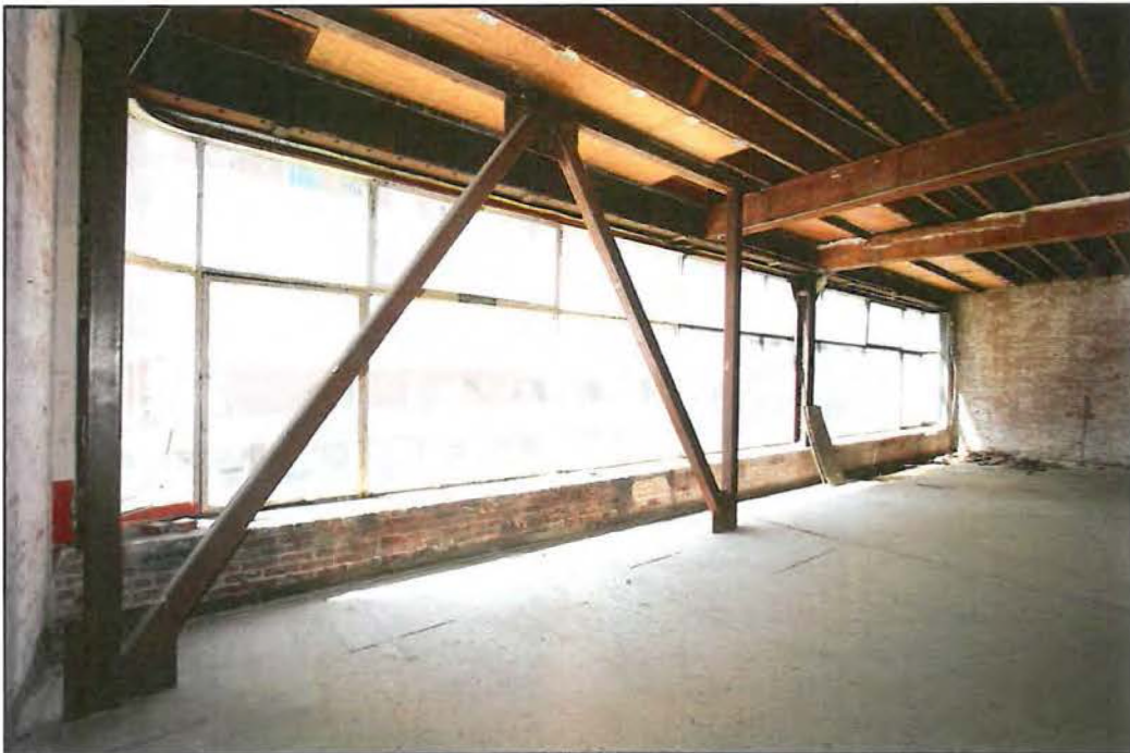
Figure 90: Second story windows facing west (Chattel, 2015).
