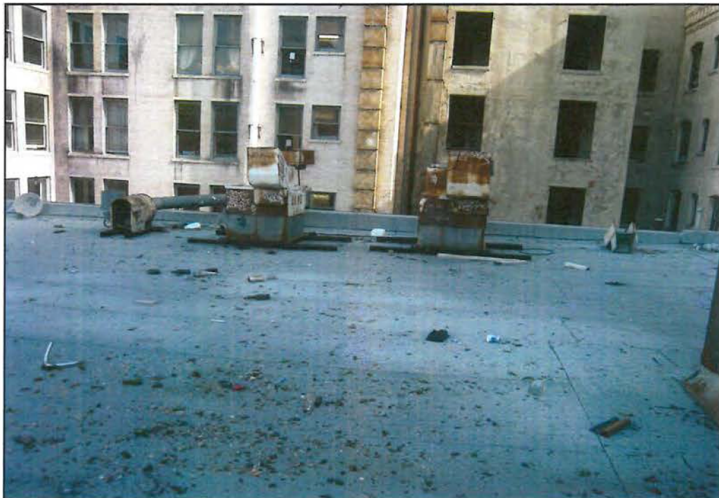
Figure 109: View of the roof, facing north (Chattel, 2015).
