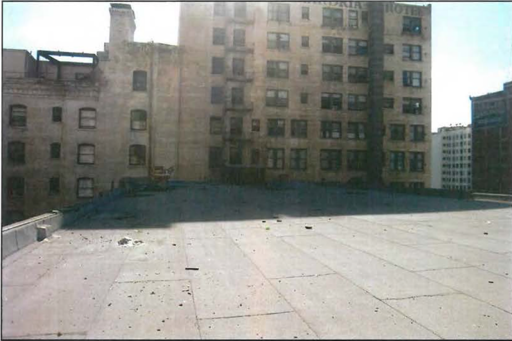
Figure 110: Roof, facing east (Chattel, 2015).
