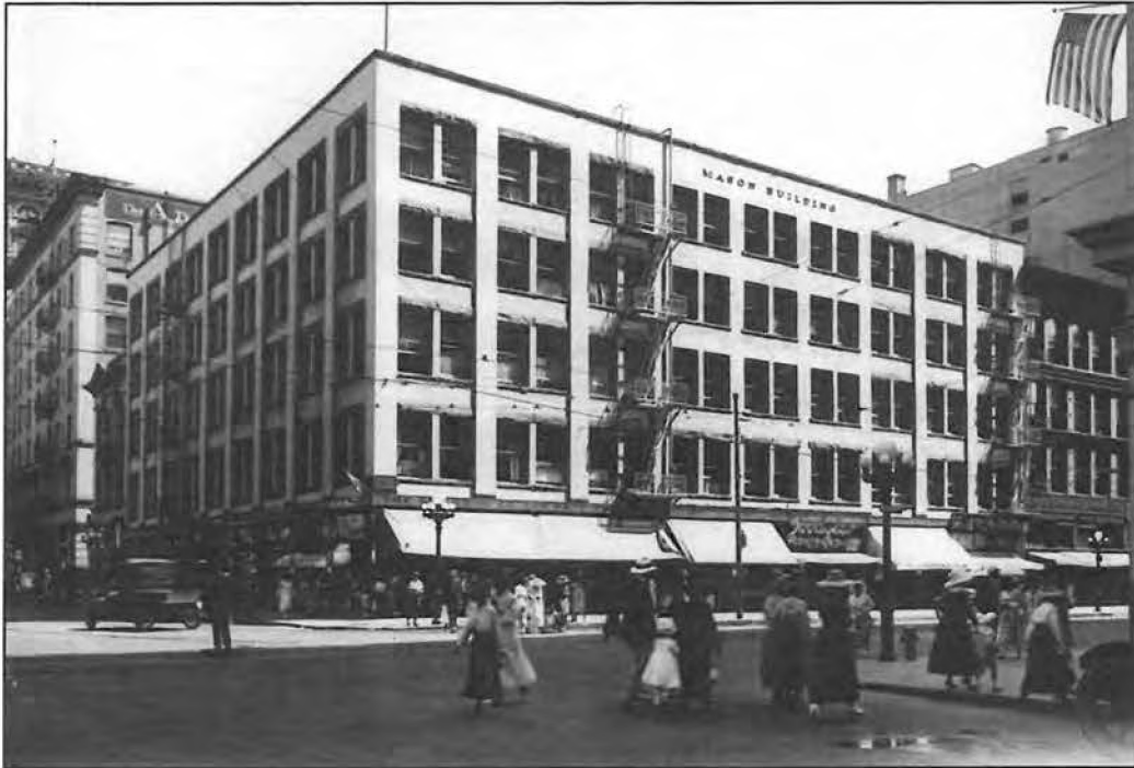
Figure 58: A view of the Mason building at the southeast corner of 4th and Broadway, designed by Robert B. Young (Los Angeles Public Library Digital Archives, Security Pacific National Bank Collection, n.d).
