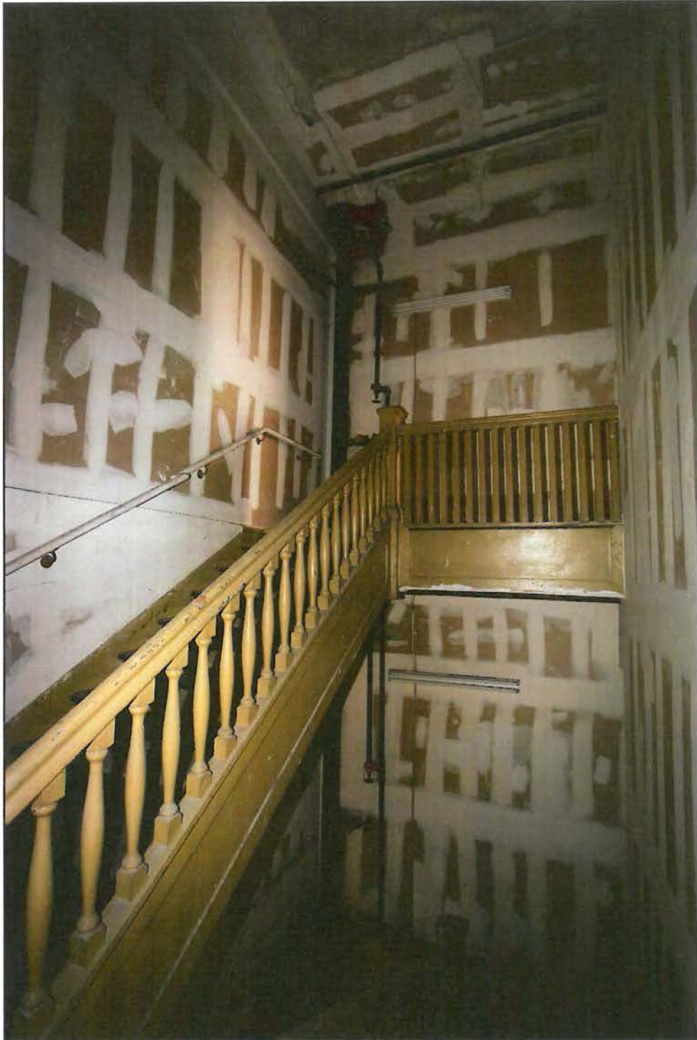
Figure 97: Staircase between second and third floor (Chattel, 2015).
