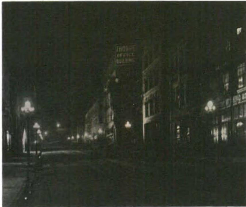
Figure 20: Photograph of Broadway's new lighting system, designed by an employee of the Forve-Pettebone Company (Underwood, 1906).
