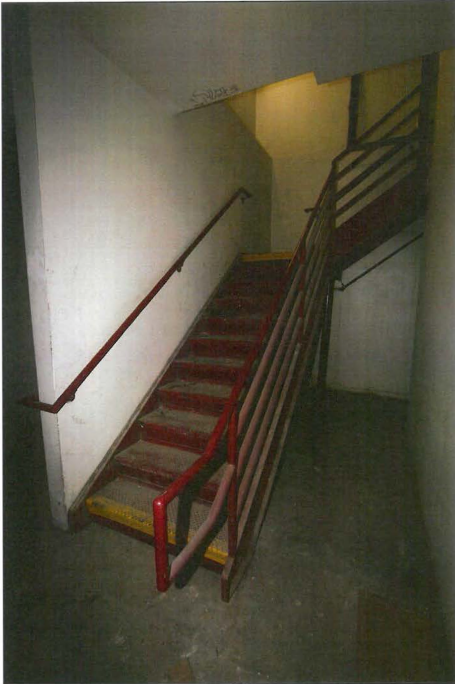
Figure 78: Interior staircase leading to basement (Chattel, 2015).
