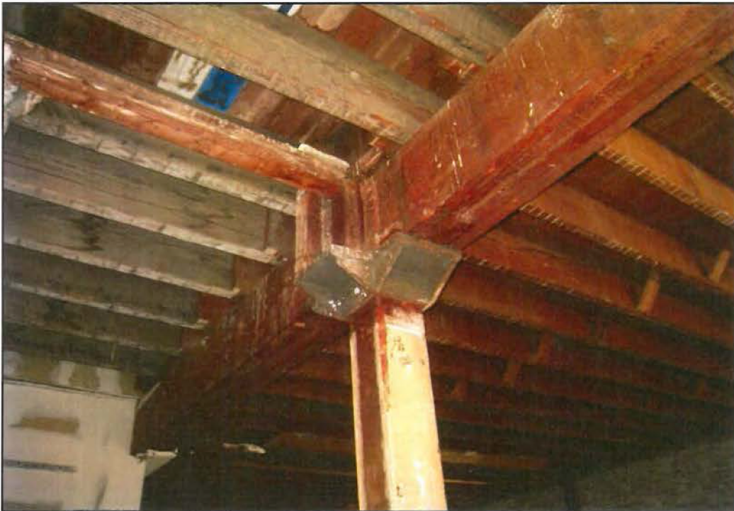
Figure 103: Detail of wood column (Chattel, 2015).
