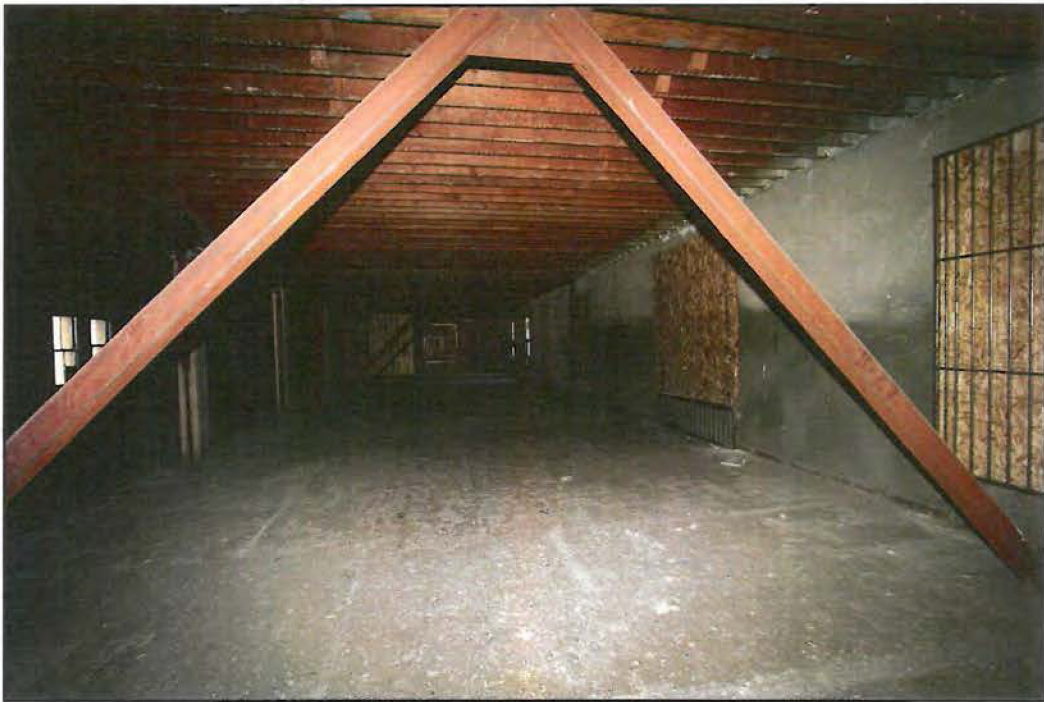
Figure 107: Interior of fifth floor, facing east (Chattel, 2015).
