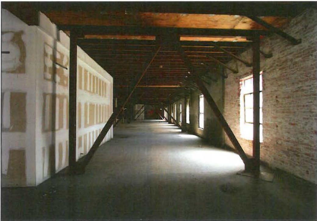
Figure 94: Second floor interior facing east (Chattel, 2015).
