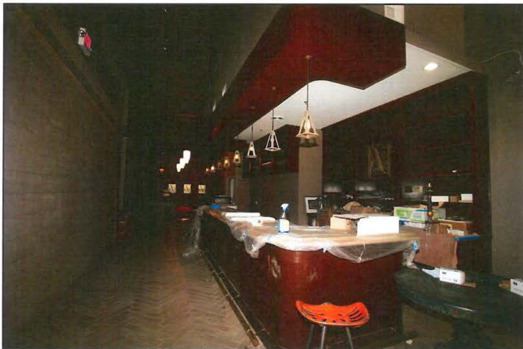
Figure 85: Interior of the current restaurant renovations at 510 South Broadway (Chattel, 2015).
