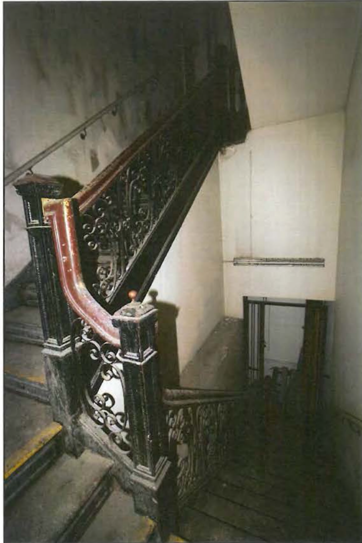
Figure 88: Interior staircase leading from ground floor to second story (Chattel, 2015).
