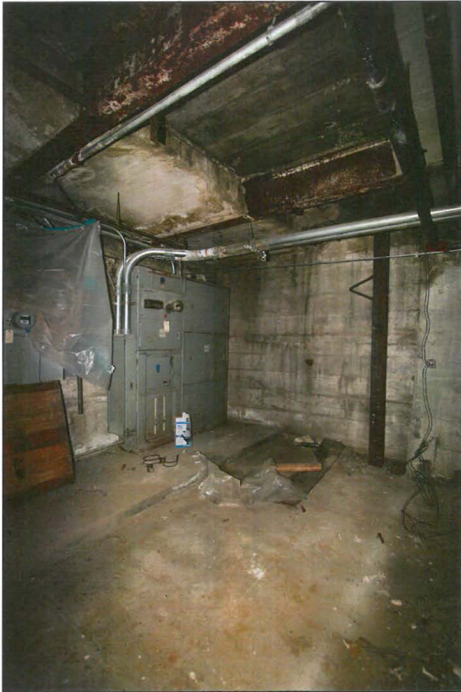
Figure 81: Sidewalk vault, facing west from the interior of the basement (Chattel, 2015).
