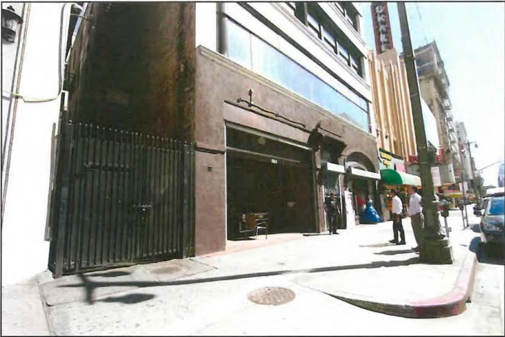
Figure 72: Oblique view of the west elevation and storefronts (Chattel, 2015).
