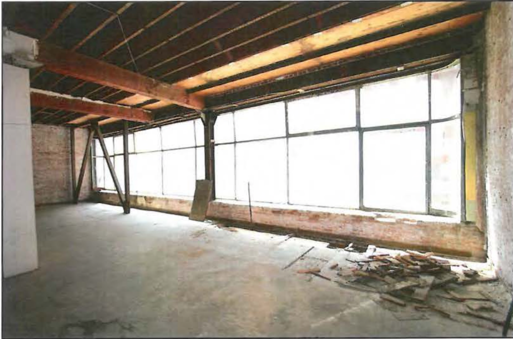
Figure 89: Second story windows facing west (Chattel, 2015).
