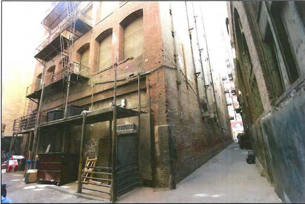
Figure 75: Oblique view of north and east elevations, and northern alley (Chattel, 2015).
