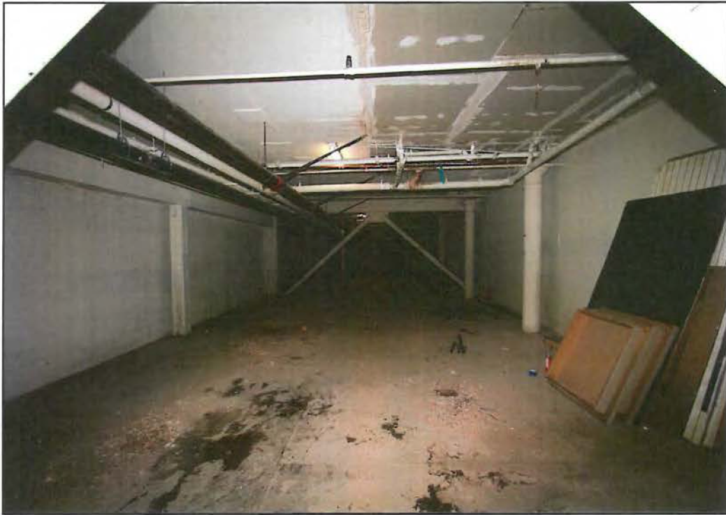
Figure 79: Interior of basement, with original cast iron columns (Chattel, 2015).
