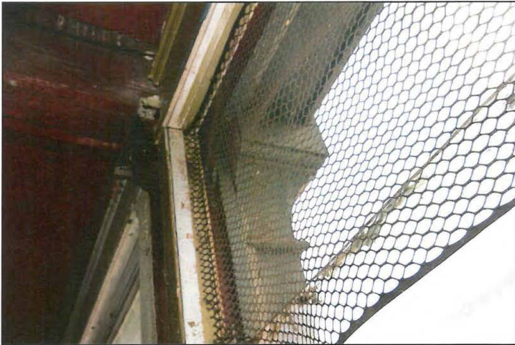
Figure 106: Interior of fifth floor windows, facing west (Chattel, 2015).
