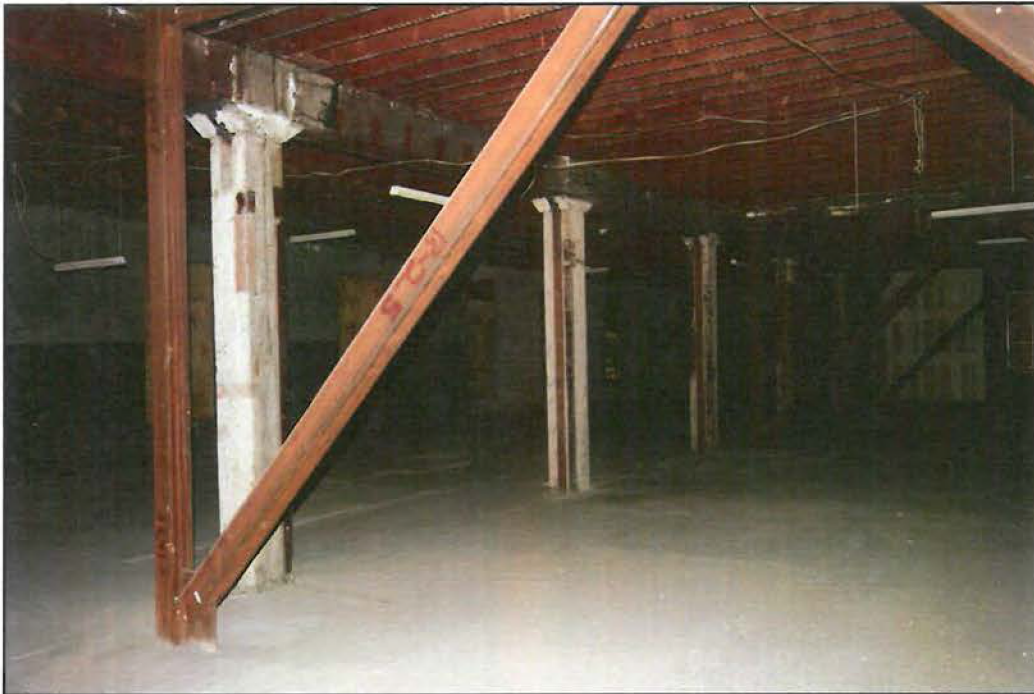
Figure 95: Interior of second floor, facing northeast (Chattel, 2015).
