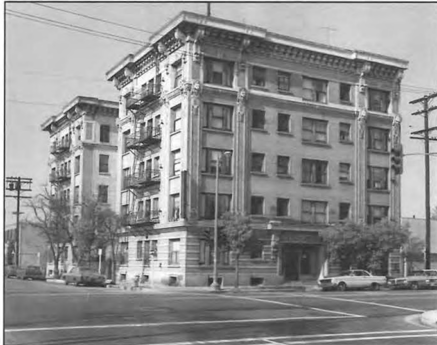
Figure 61: Young Apartments, 1615-1631 South Grand Avenue, designed by Robert Brown Young & Son (firm) in 1912. This property is a Historic-Cultural Monument #317 and has been determined eligible for the National Register of Historic Places. (Los Angeles Public Library Digital Archive, 1972).
