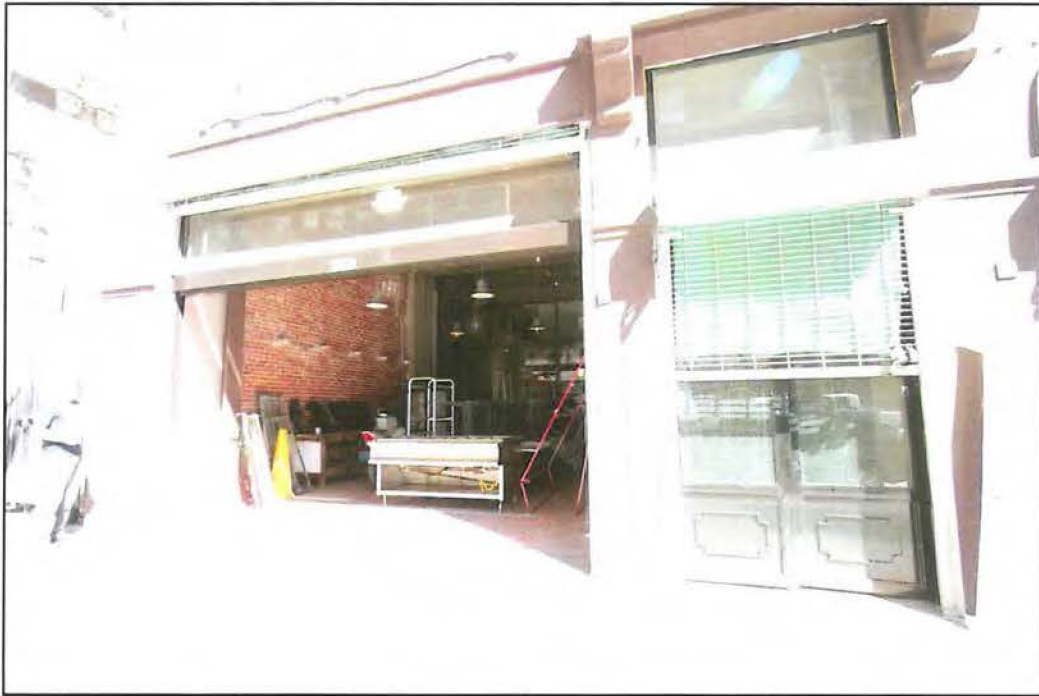
Figure 82: Exterior of 510 South Broadway storefront and main entrance (Chattel, 2015).
