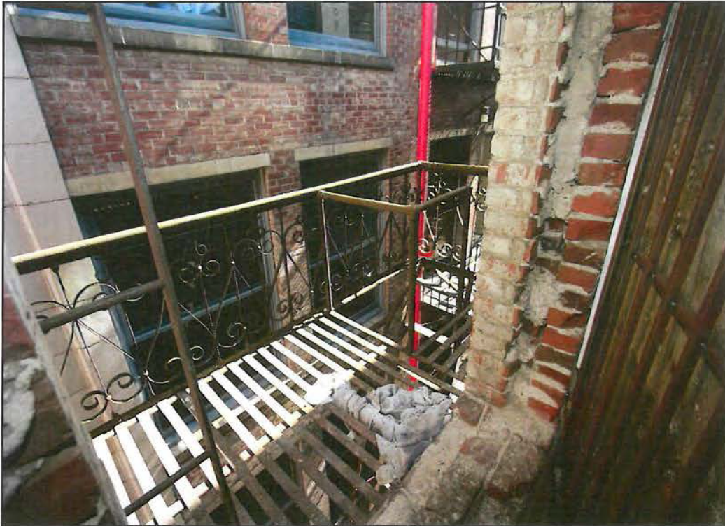
Figure 108: Exterior of fifth floor, north elevation fire escape (Chattel, 2015).
