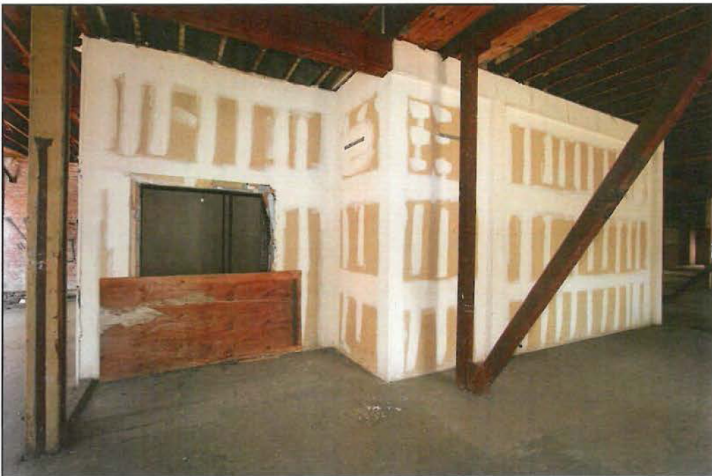
Figure 96: Elevator shaft, second floor (Chattel, 2015).
