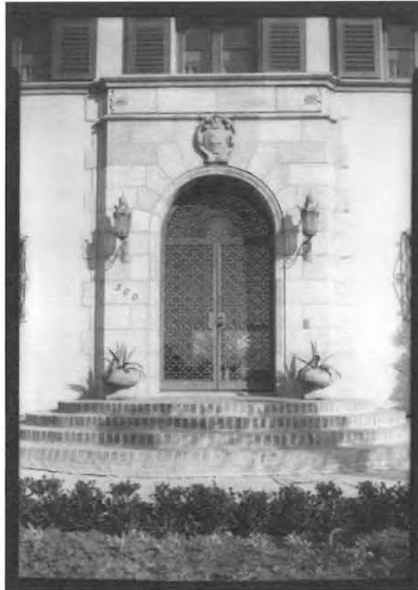
Figure 29: Exterior of 500 South Hudson Avenue, fixtures designed by Forve-Pettebone Company (Dick Whittington, USC Digital Library, 1926.).
