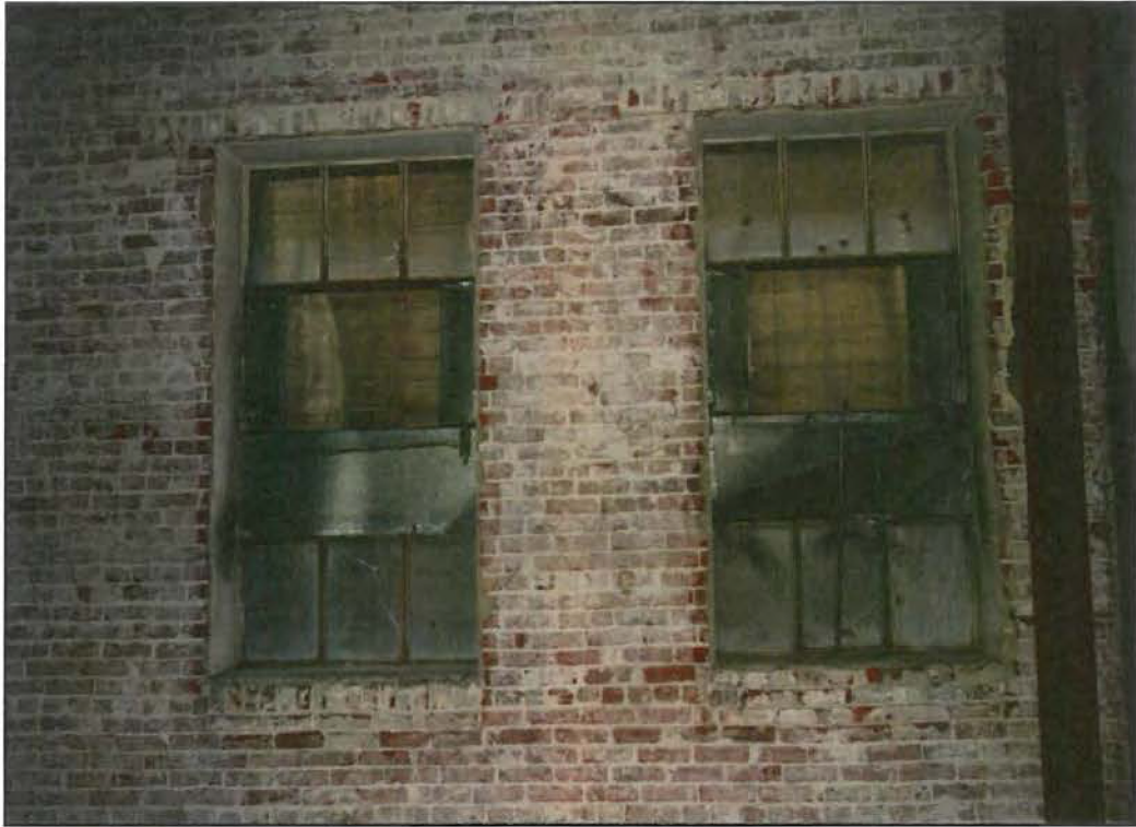
Figure 104: Pair of windows on fourth floor, north elevation (Chattel, 2015).
