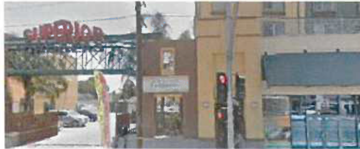
Superior Market Development as First Floor Retail of New Affordable Housing @ 2000 S. Central Avenue, LA 90011
