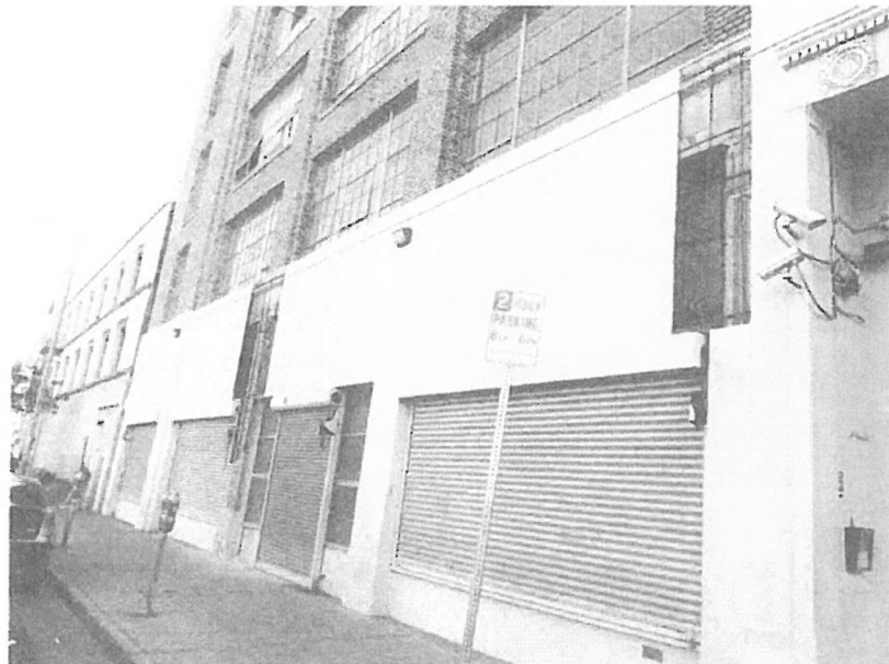
The new owner is planning a rehabilitation of the building including the façade. Recent investigations have revealed that the original façade exists under the current material. Plans are being prepared by the architect for the project and façade restoration. This photo shows the two areas that were exposed.
