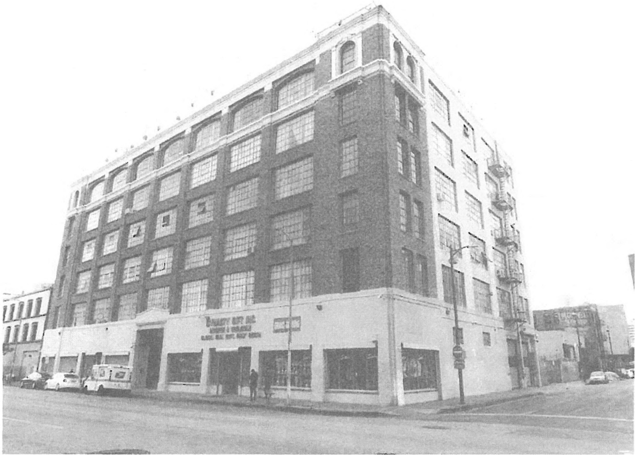
Catalina Swimwear Building, Primary façade (east) and secondary (north) elevation. The building is highlighted and characterized by Neoclassic detailing on the sixth floor. The first story of the façade is furred out, obscuring the original terra cotta pilasters which survive behind the stucco.
