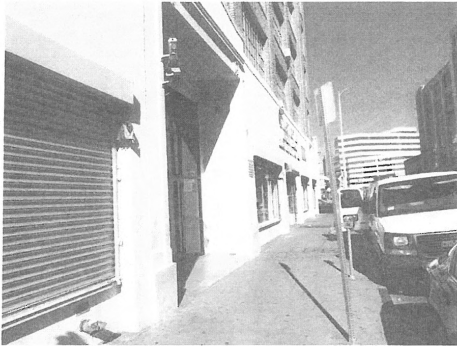
Original 1923 Entrance, and storefront modified in 1960 by furring out over original material.
