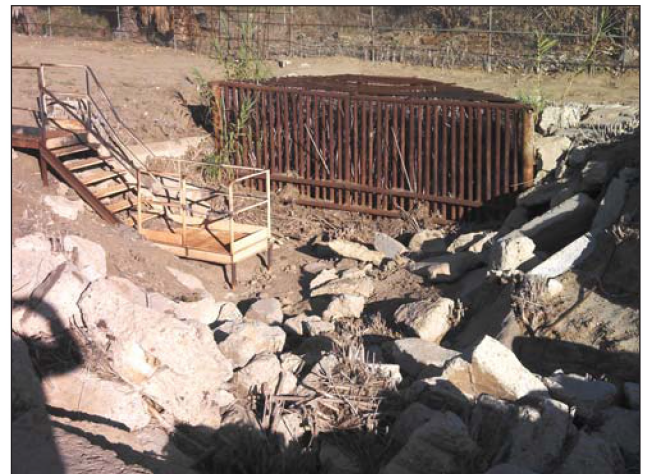
Looking north at the storm drain inlet at the northeastern corner.
