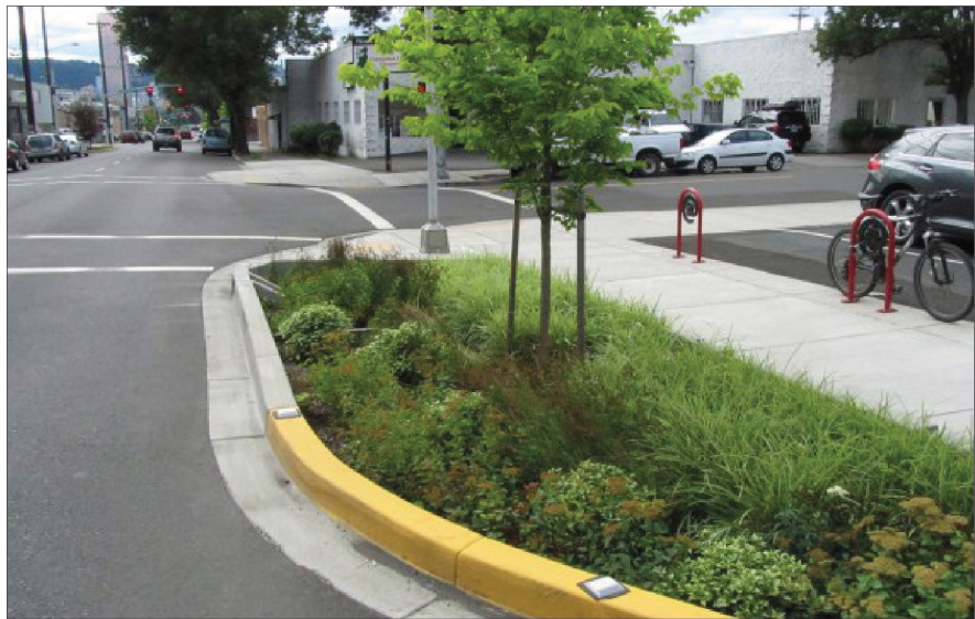
Corner curb extension with optional planting
