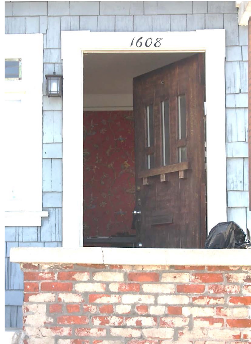
South original entry on west façade with original brick wall, door partially open, view east.
