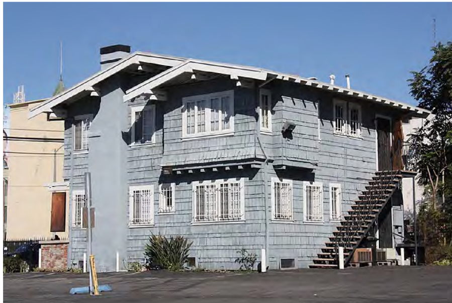
South elevation with unusual feature in south wall of second level extended gable which wraps beyond frame of residence into east elevation, providing space for the original dining room breakfront with window at either side. Second level paired multi-pane casements, exit with replacement stairs. Ground floor paired/single multi-pane casements, exit/utilities beneath stairs, crawl space vents, view northwest.
