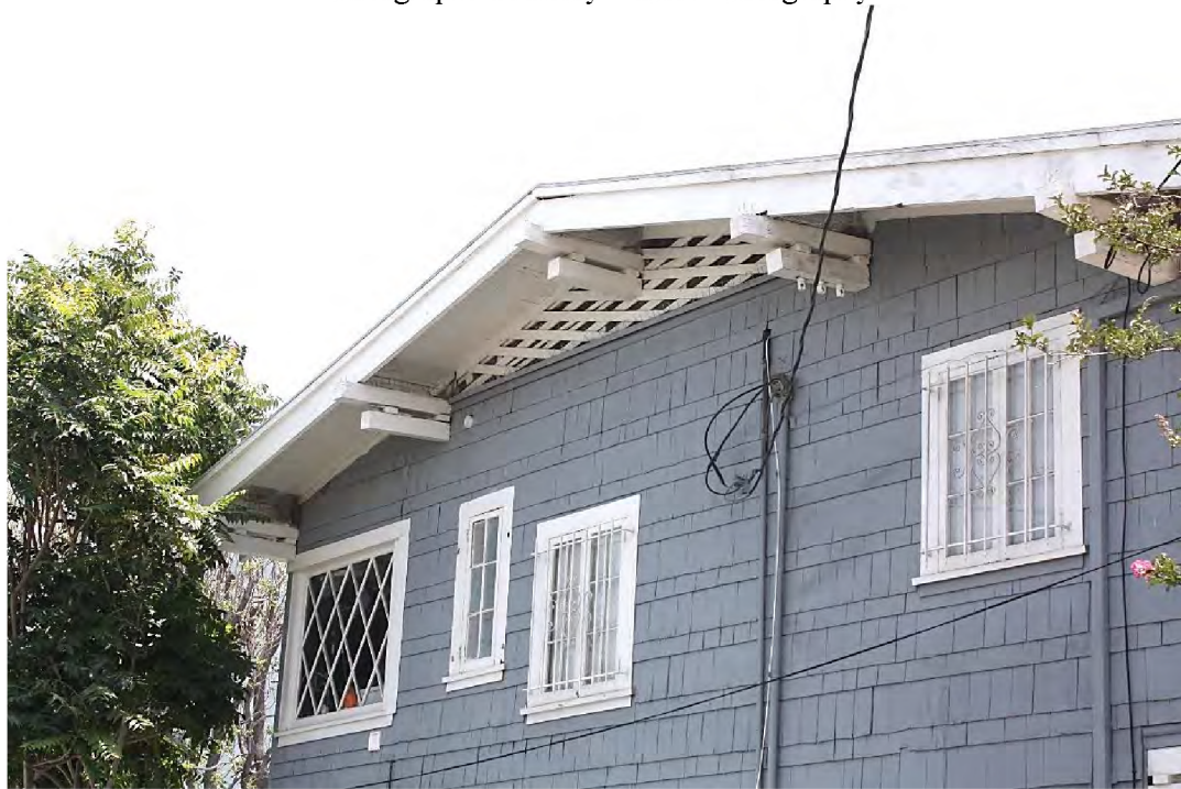
Detail, north elevation: Broad eave, criss-cross vent, decorative double beam ends. Diamond pane picture window; single, & paired 6-pane casement windows, view southeast. Photograph: Courtesy Michael Medina.
