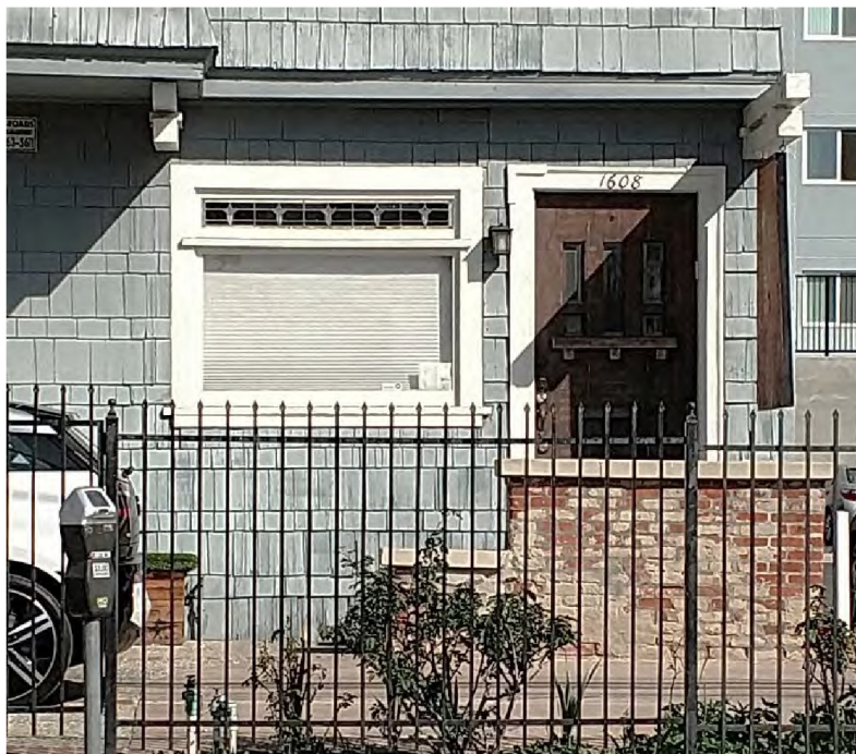
1608 N. Las Palmas: Window, entry, view east.
