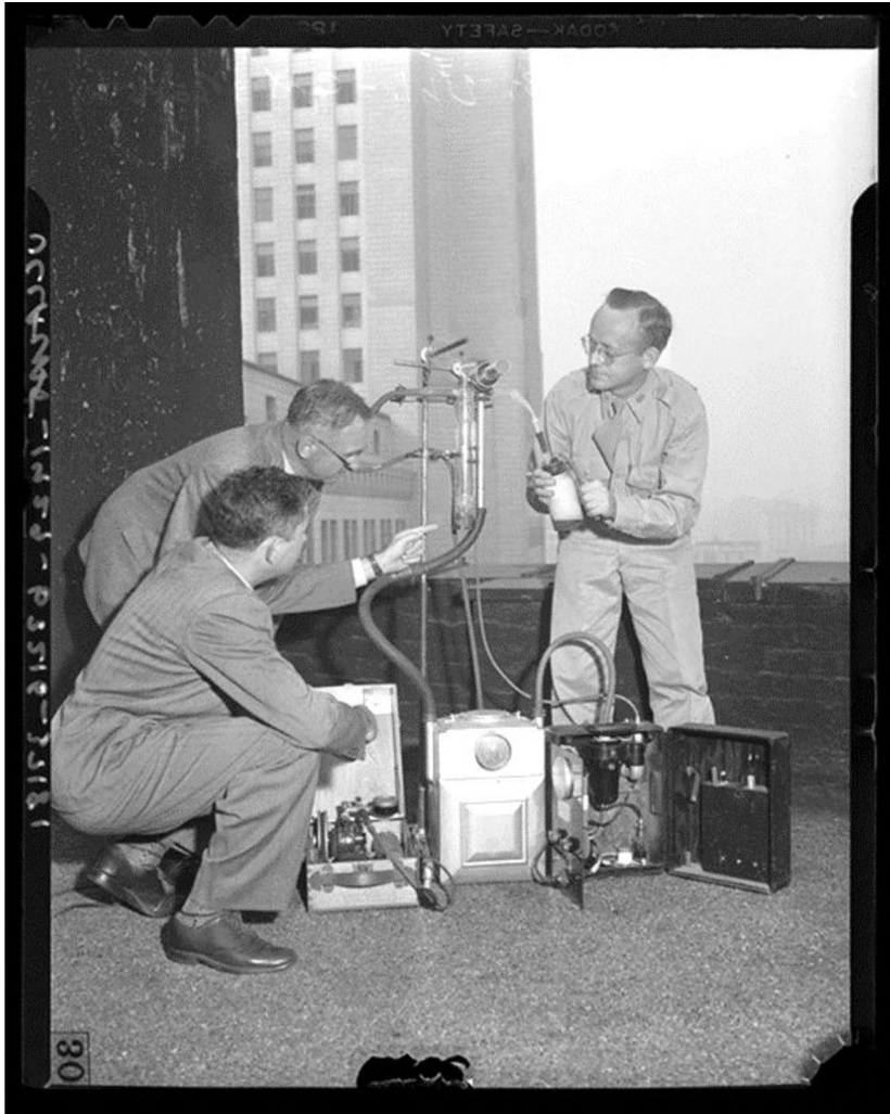
Smog Catcher: Left to right, Dr. George M. Uhl, city health officer, pointing; Harry E. Kunkel and Capt. Thomas Marsh demonstrating electrostatic precipitator, or "smog catcher." Actual photograph, same ran in the Los Angeles Times, Sept 14, 1945, page A1.
