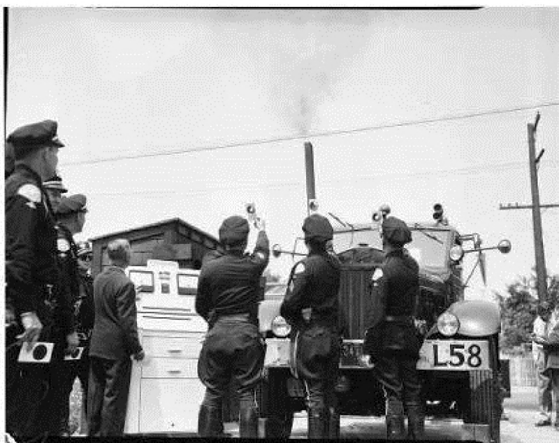
Harry E. Kunkel, (City Air Pollution Control Officer) demonstrating a new smog detector on a diesel truck, while motorcycle officers who would ride “smog snoopers” patrols, as they were referred to by Kunkel, observe. June 1947, Los Angeles Examiner Negatives Collection, USC Digital Library.
