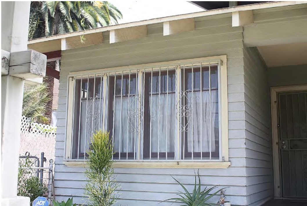
Detail: Four casement windows with paired transoms at west façade. North corner is representative of all windows in the residence.
