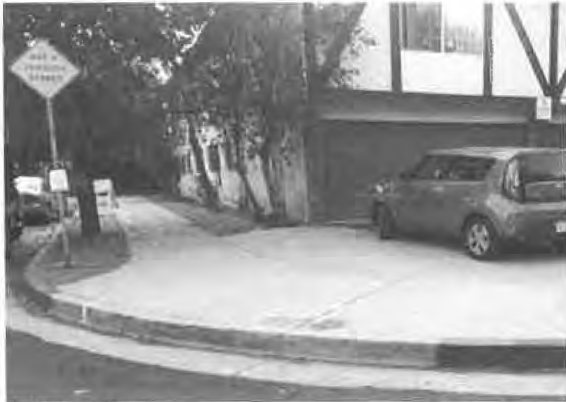
Curb Ramp Needed
